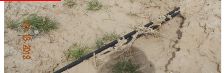
Photo#4: Wash out of ditch & rocked drain has occurred.
