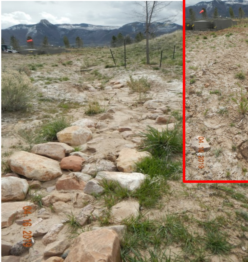
Photo#3: Wash out of ditch & rocked drain has occurred
