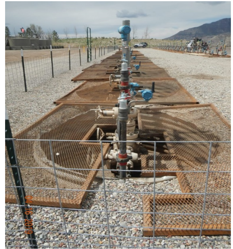
Photo#2: There are no Wildlife escape boards installed in Well Cellars.
