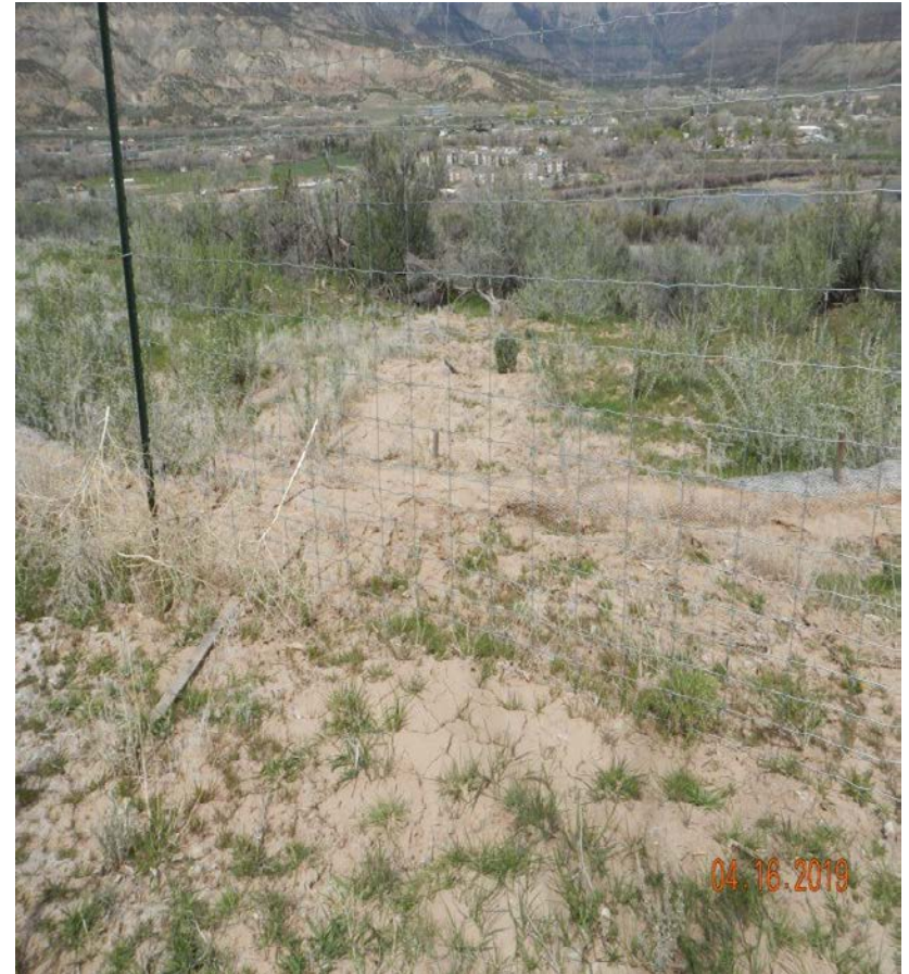
Photo#6: Sediment moving through perimeter fence, overwhelming wattles and migrating off site.
