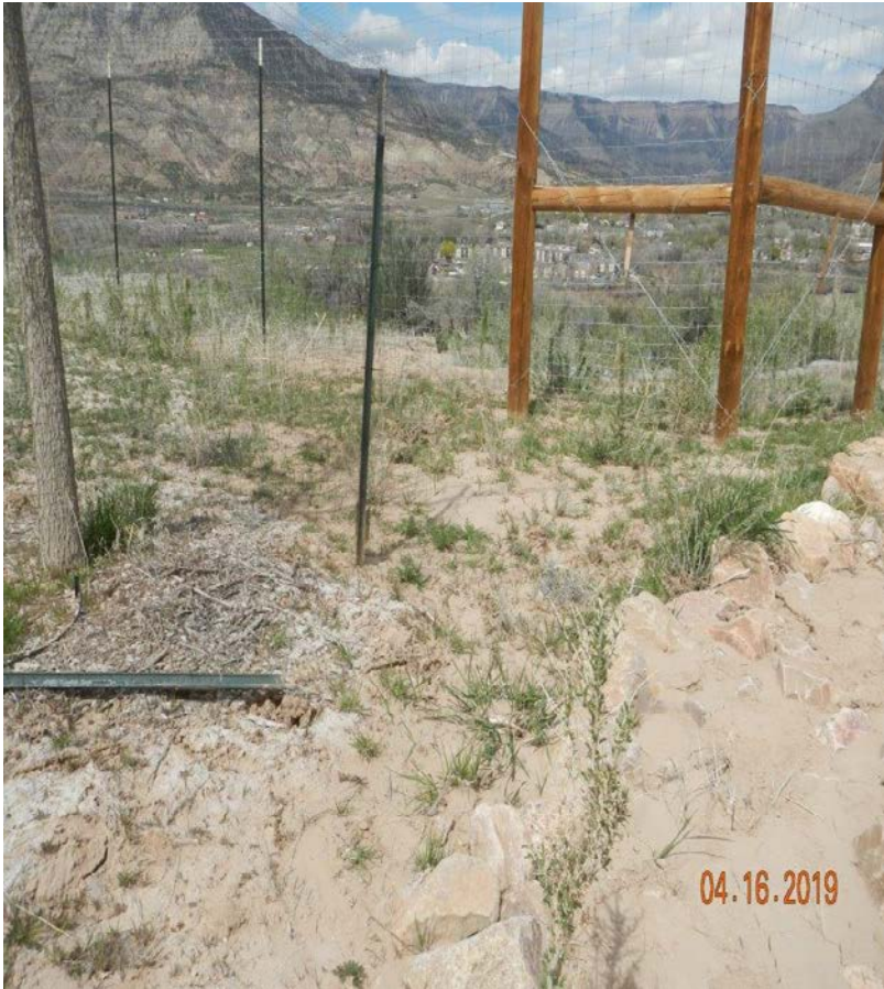
Photo#5: Sediment moving through perimeter fence, overwhelming wattles and migrating off site.
