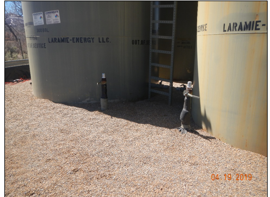
Photos of risers not locked out or tagged
