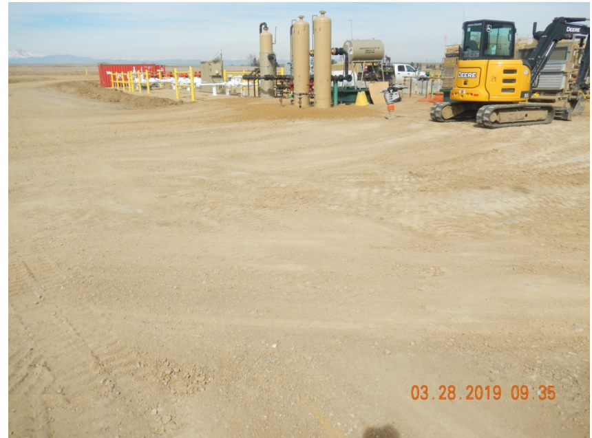
Photo 8. Photo taken from the northeastern perimeter of the location, facing West. No silt traps with stabilized outlets were observed on location.
