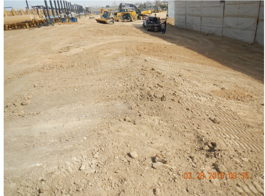
Photo 6. Photo taken from the eastern perimeter of the location, facing North. The ditch and berm BMP does not go around the entire perimeter of the location.
