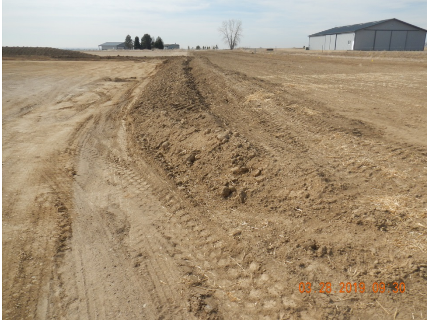
Photo 1. Photo taken from the northwestern perimeter of the location, facing South. Photo illustrates a compacted BMP that has been installed around parts of the location.
