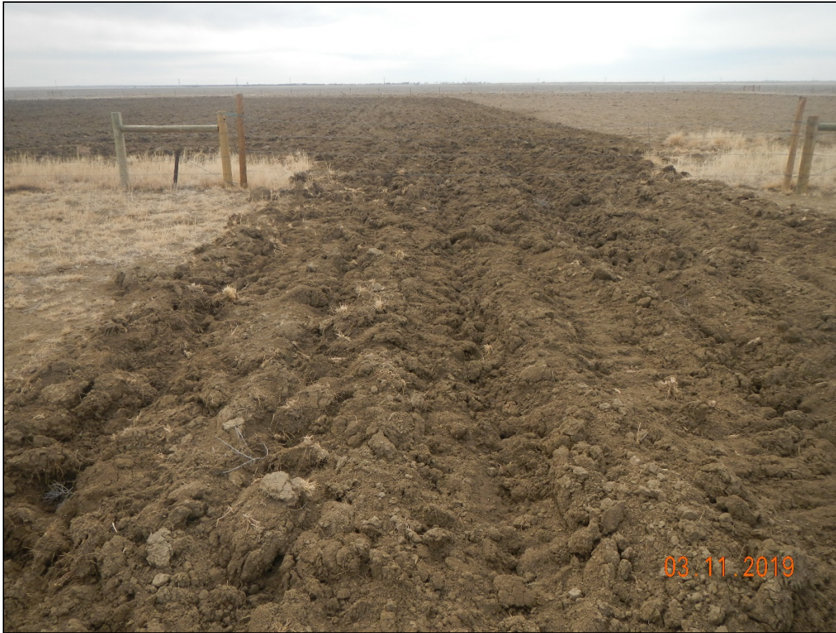
Photo 4. Facing toward the location. Decompaction has occurred at the location.
