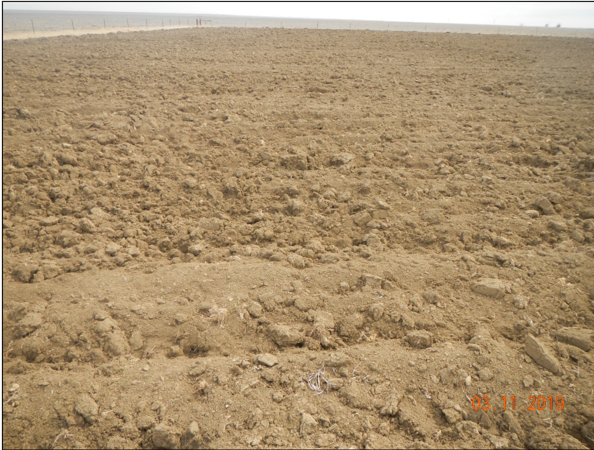
Photo 5. Facing east at the location. Soil decompaction has occurred at the location. The soil has not been seeded and stabilized.
