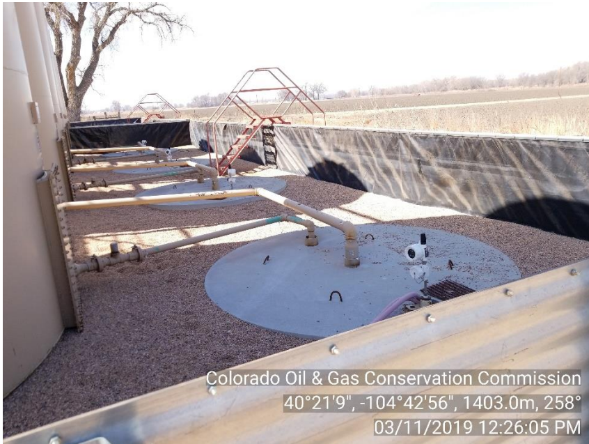
Photo 5: No visible securing mechanism on produced water tanks.
