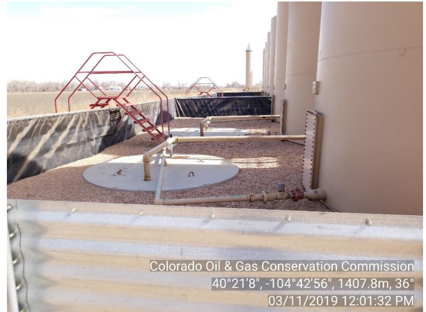
Photo 4: No visible securing mechanism on produced water tanks.
