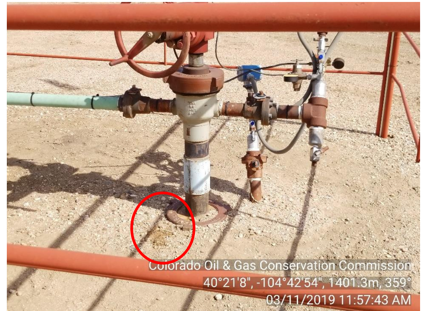
Photo 2: Stained soil at main valve.
