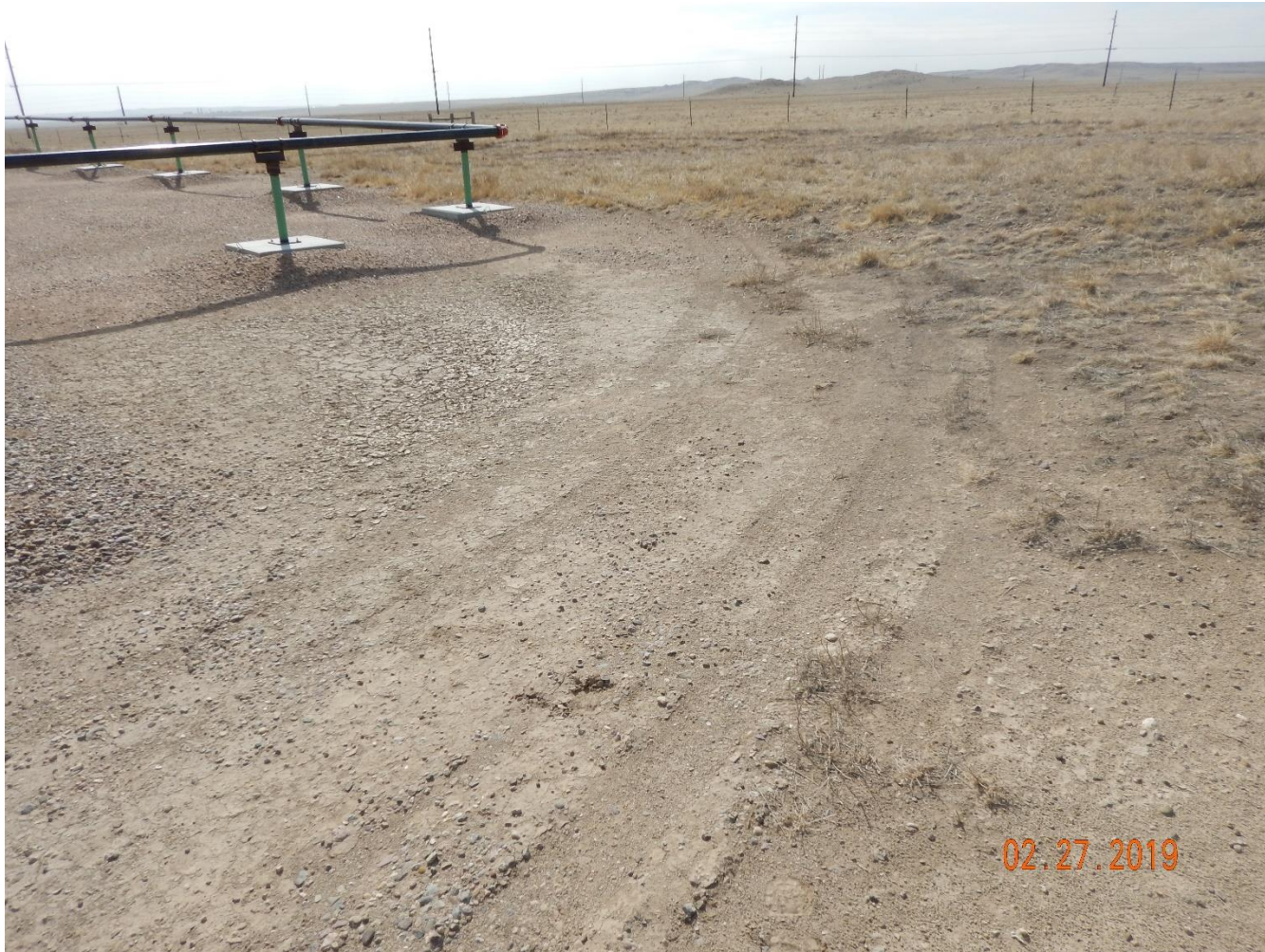
Photo 4: Photo taken from the northwest end of the pad, facing southwest. Photo shows operator appears to have traveled off of the designated pad onto the interim areas. This is not compliant with rules 1002.e. Restrict all equipment and vehicle traffic to the constructed pad and designated access road.
