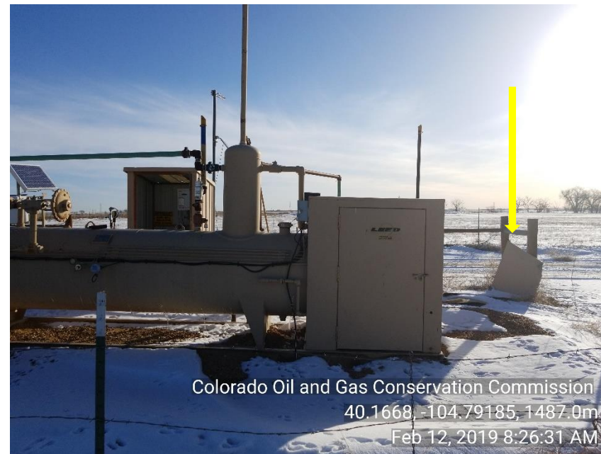
Photo 4 Trash door off meter house
