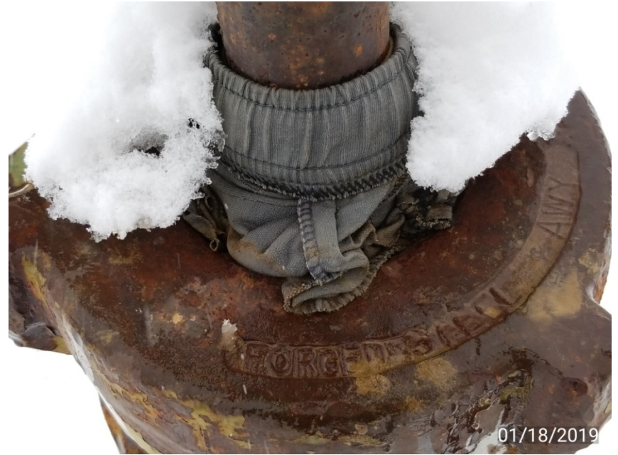
Photo 2. Well head leaking gas.
