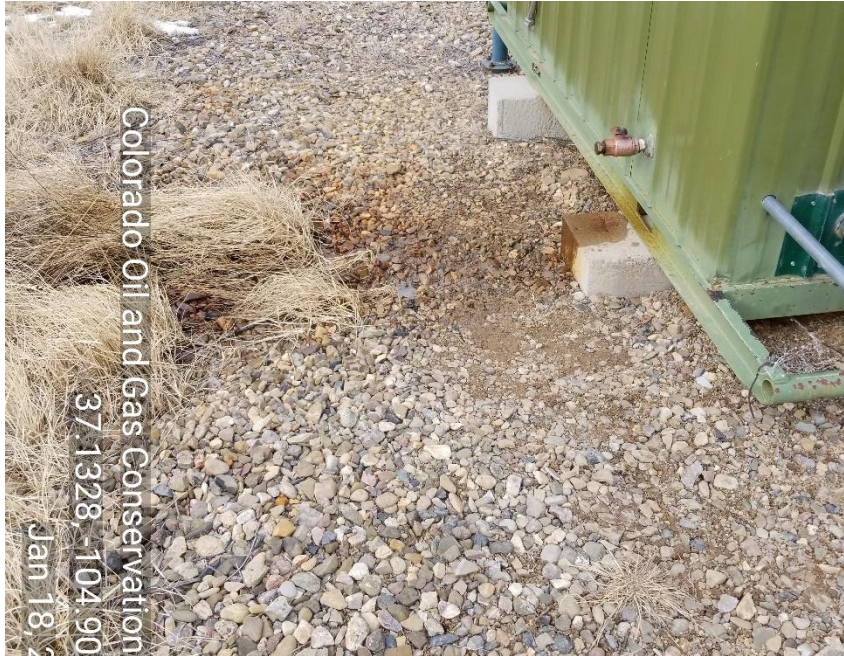
Photo 1 stained soil under 1" line to drain for separator
