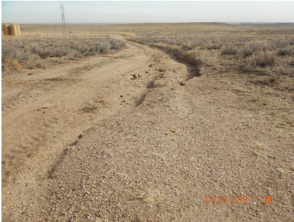
Photo 4. Photo taken from the former well location access road, facing East. Operator shall repair erosion along the access road. Note: the gravel that has been washed eastward was likely from the well location.
