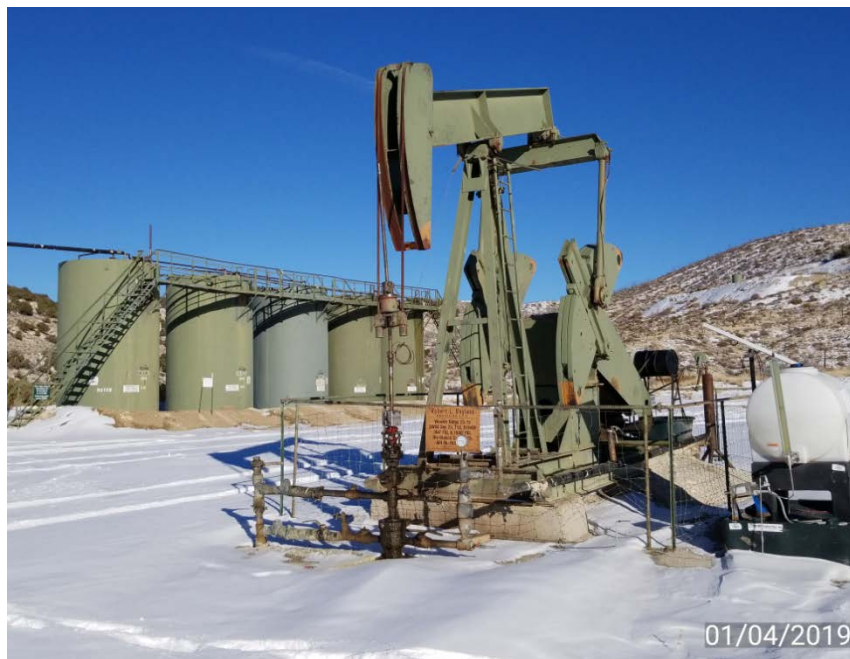
Photo 3. Pump jack and tank battery.
