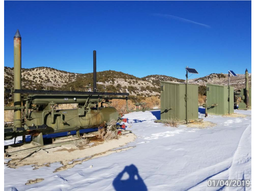
Photo 2. Separators and gas meter buildings.
