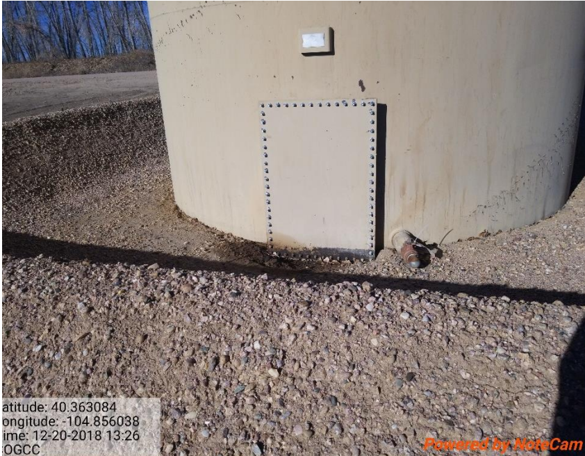
Photo 3 – Staining at crude tank access.
