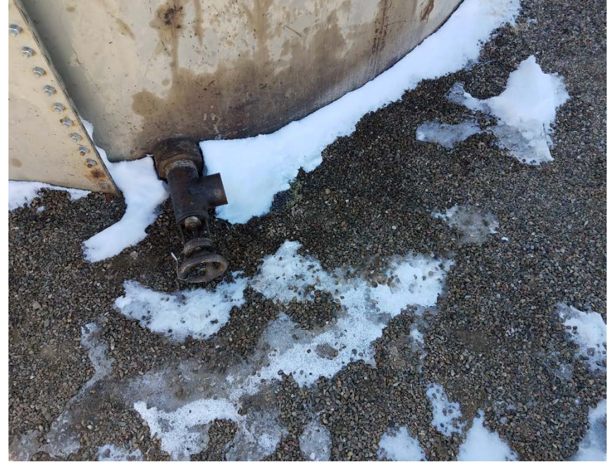
Location Photo #5, Oil stained rock in battery containment.
