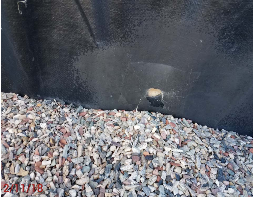
Location Photo #3, Holes in containment liner.
