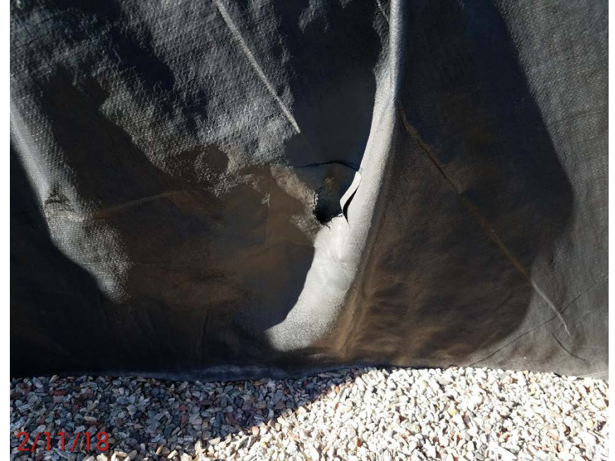
Location Photo #2, Holes in containment liner.
