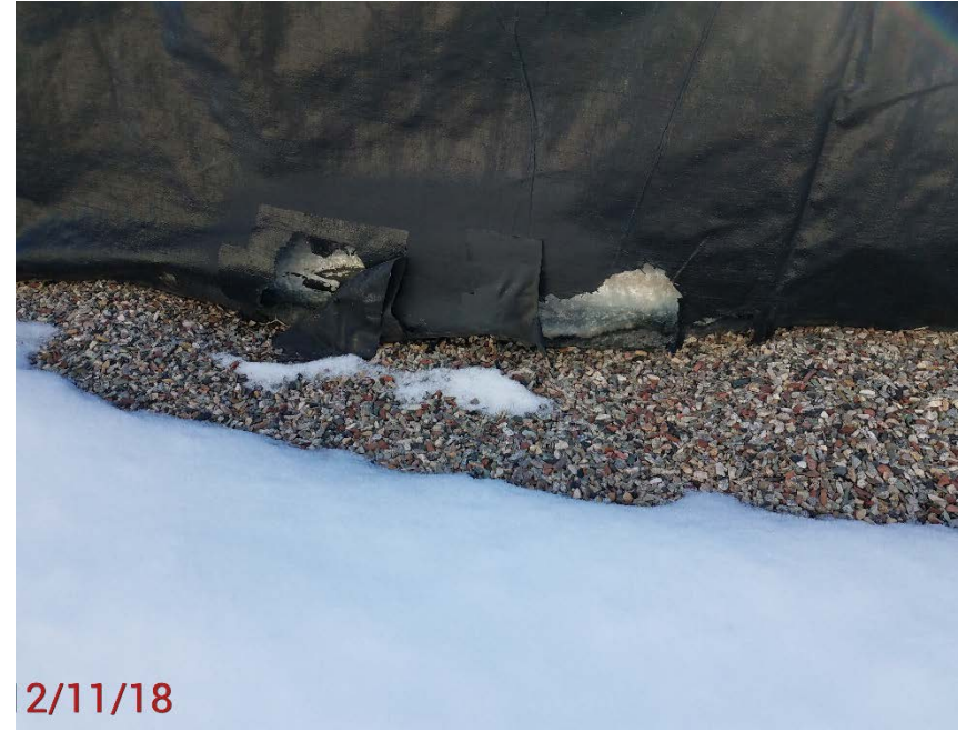
Location Photo #4, Holes in containment liner.
