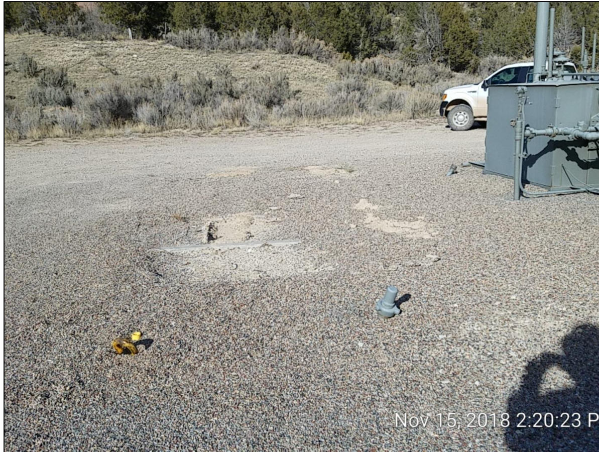
Deadman marker is broke off. Unmarked risers at separator.
