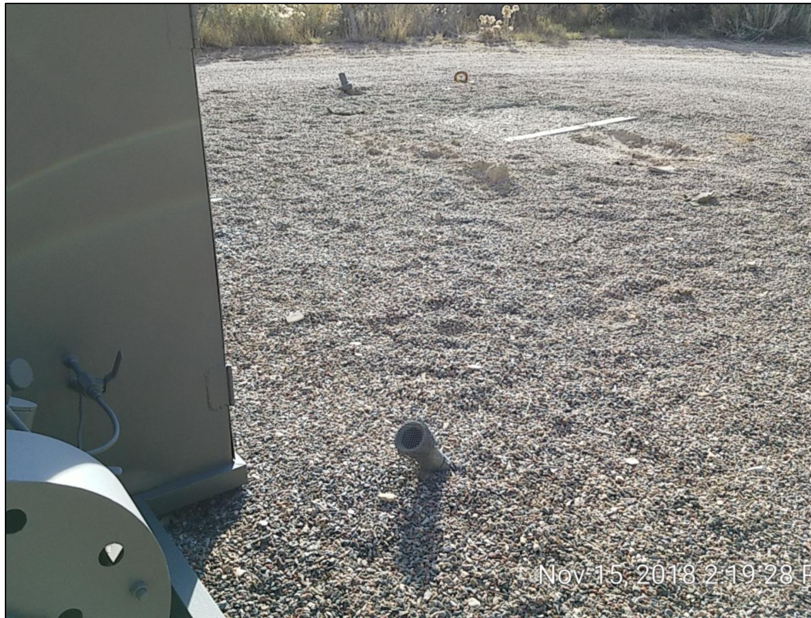
Unmarked risers at separator.
