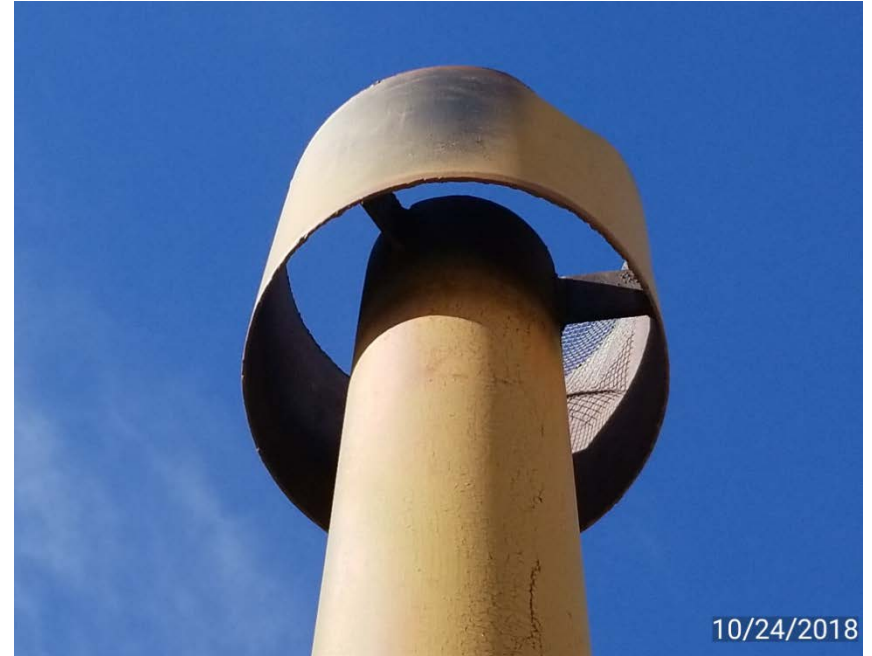
Bird screen no longer over stack opening
