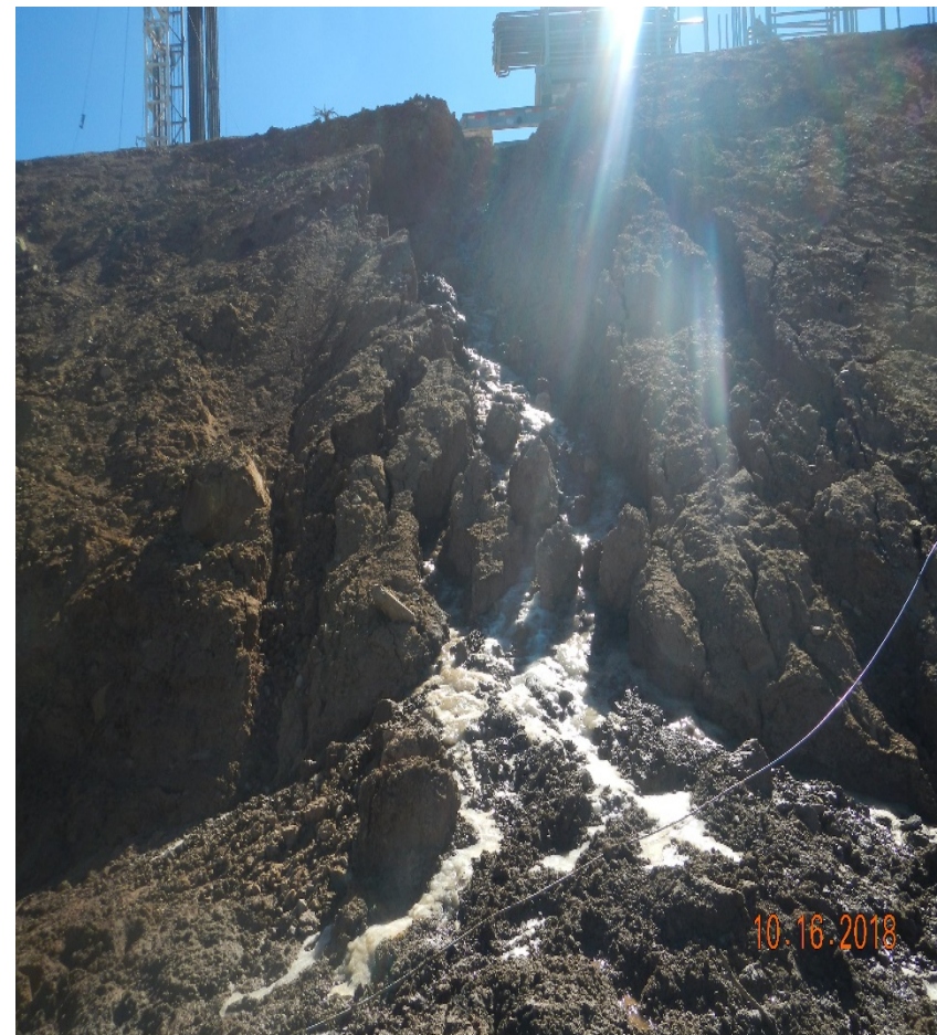
Photo#4: View from base of slope of failed BMP area.
