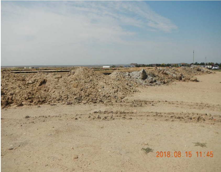
Photo 9. Spoil pile without storm-water BMPs
