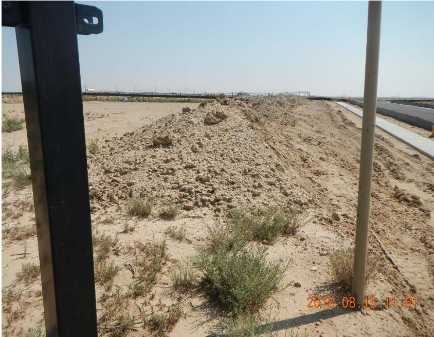
Photo 11. Perimeter fence was removed from south side of location. Spoil pile without storm-water BMPs.
