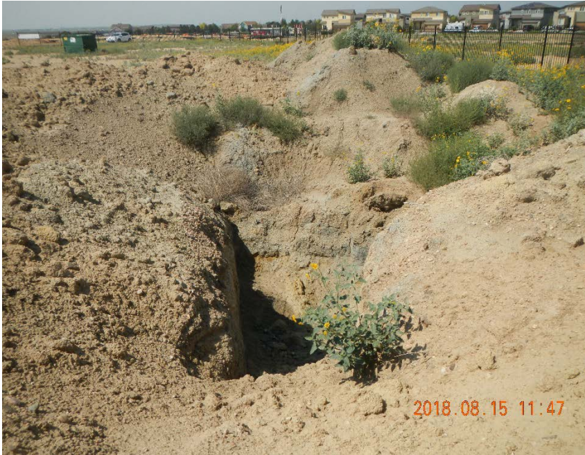
Photo 7. Open excavation without temporary safety fencing
