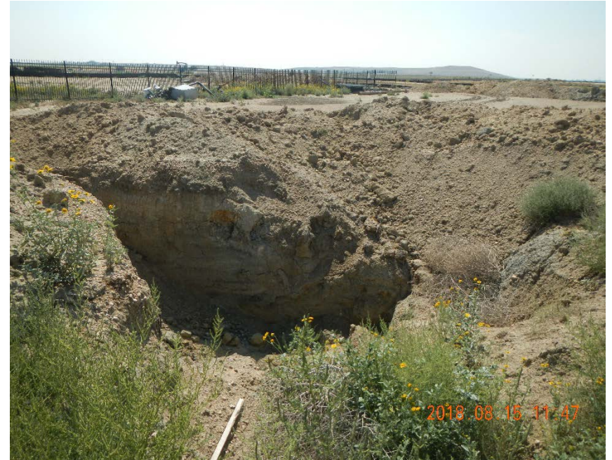
Photo 6. Open excavation without temporary safety fencing
