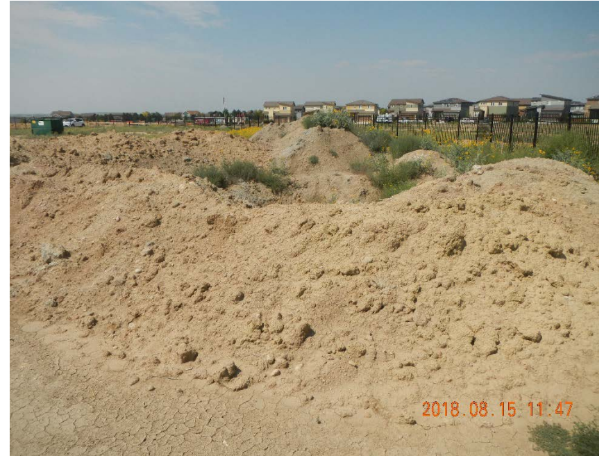
Photo 10. Spoil Pile without storm-water BMPs
