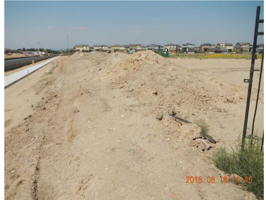
Photo 4. Spoil pile along south side of location. No storm water BMPs.
