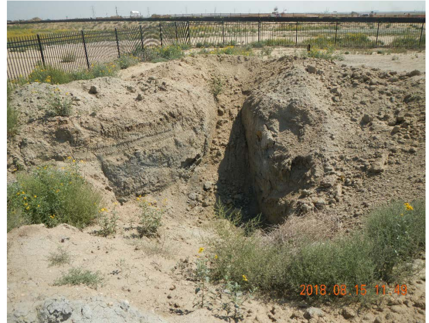
Photo 8. Open excavation without temporary safety fencing
