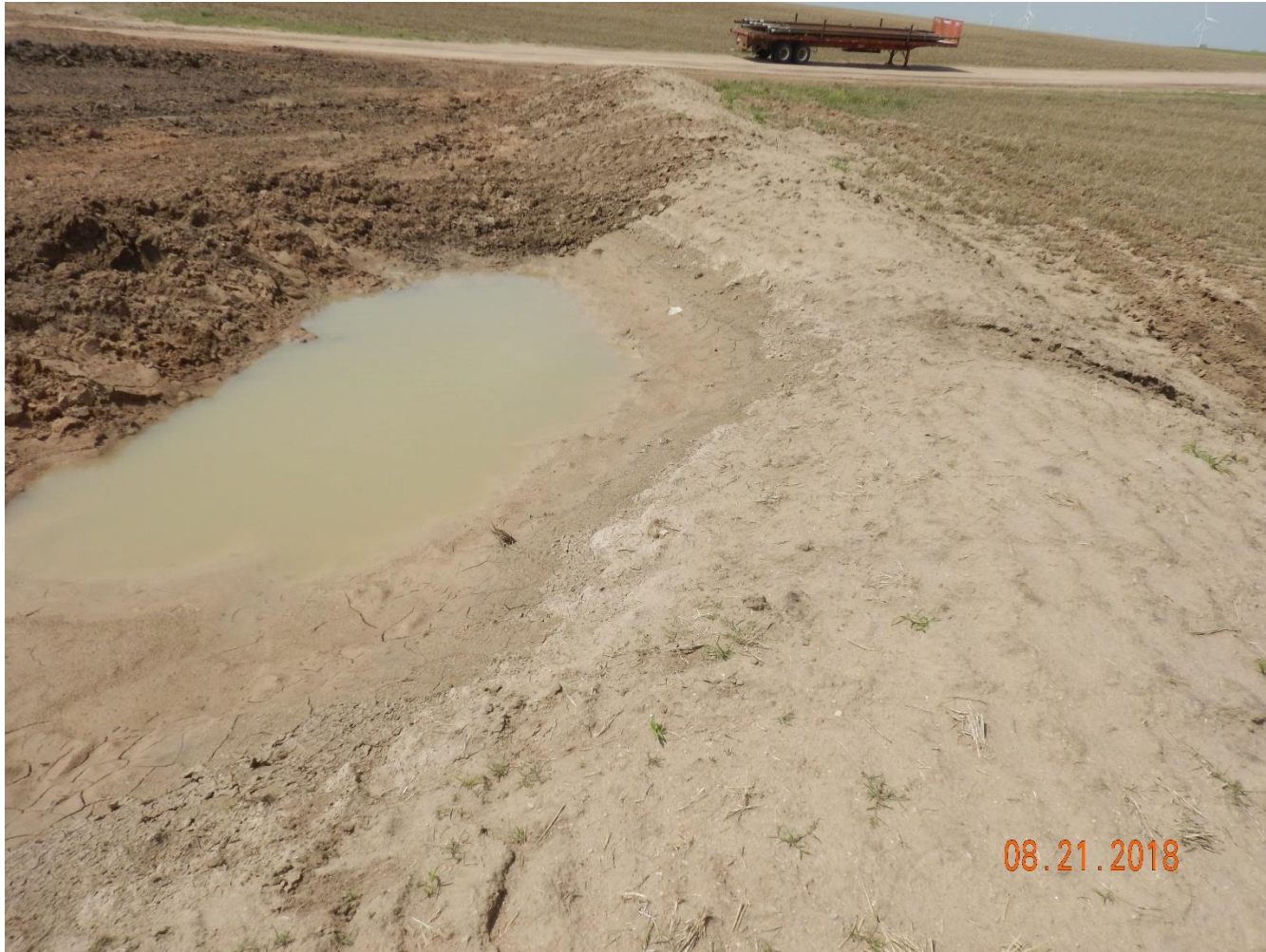
Photo 8: Photo taken from the north end of the location, facing west. Operator appears to have implemented a sediment trap, or retention pond on the southern end of the location. BMP does not appear to be appropriate in size to mitigate runoff from the 4.26 acre location. Trap/pond missing sufficient inlet and outlet protection and does not appear to be designed in such a manner to allow for sediment-laden free stormwater discharge from the location; BMP does not appear to have been constructed in accordance with good engineering practice.
