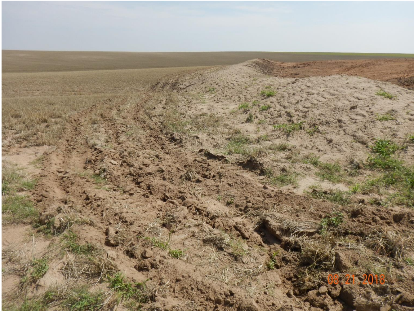
Photo 5: Photo taken from the northwest corner of the location, facing east. Photo shows stormwater and erosion control BMPs. Berm appears to have been constructed with topsoil. Berm does not appear to have been compacted, stabilized or constructed in accordance with good engineering practices. Photo also shows surface roughening along perimeter.
