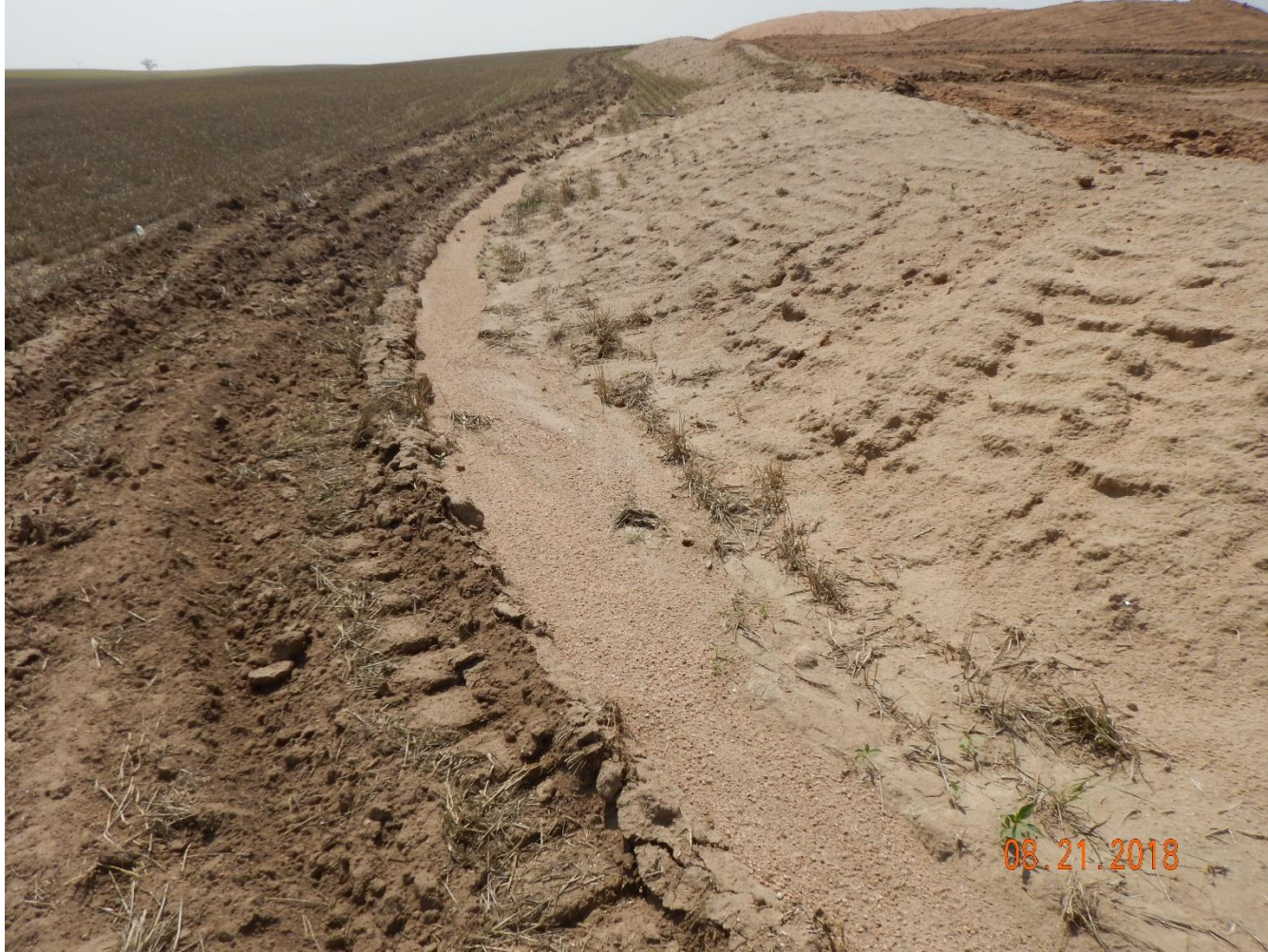
Photo 13: Photo taken from the northeast corner of the location, facing south. Photo shows erosion degradation occurring on berms as well as the resulting sediment transport and deposition. Berms do not appear to be stabilized or compacted in accordance with good engineering practices.
