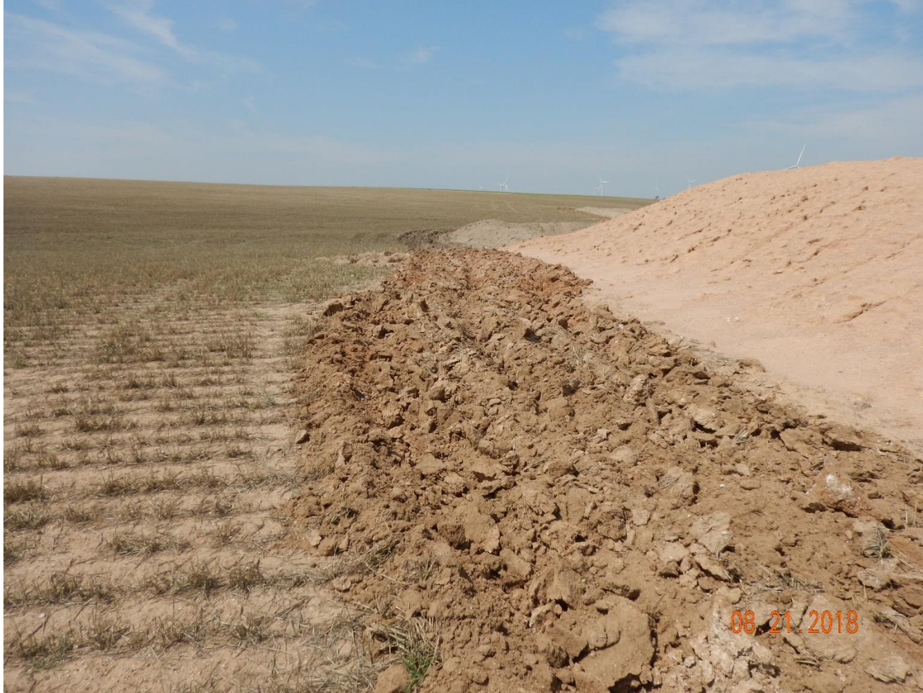
Photo 14: Photo taken from the southeast corner of the location, facing west. Photo shows surface roughening. Surface roughening is a temporary that needs to be implemented in conjunction with other stormwater and erosion control BMPs
