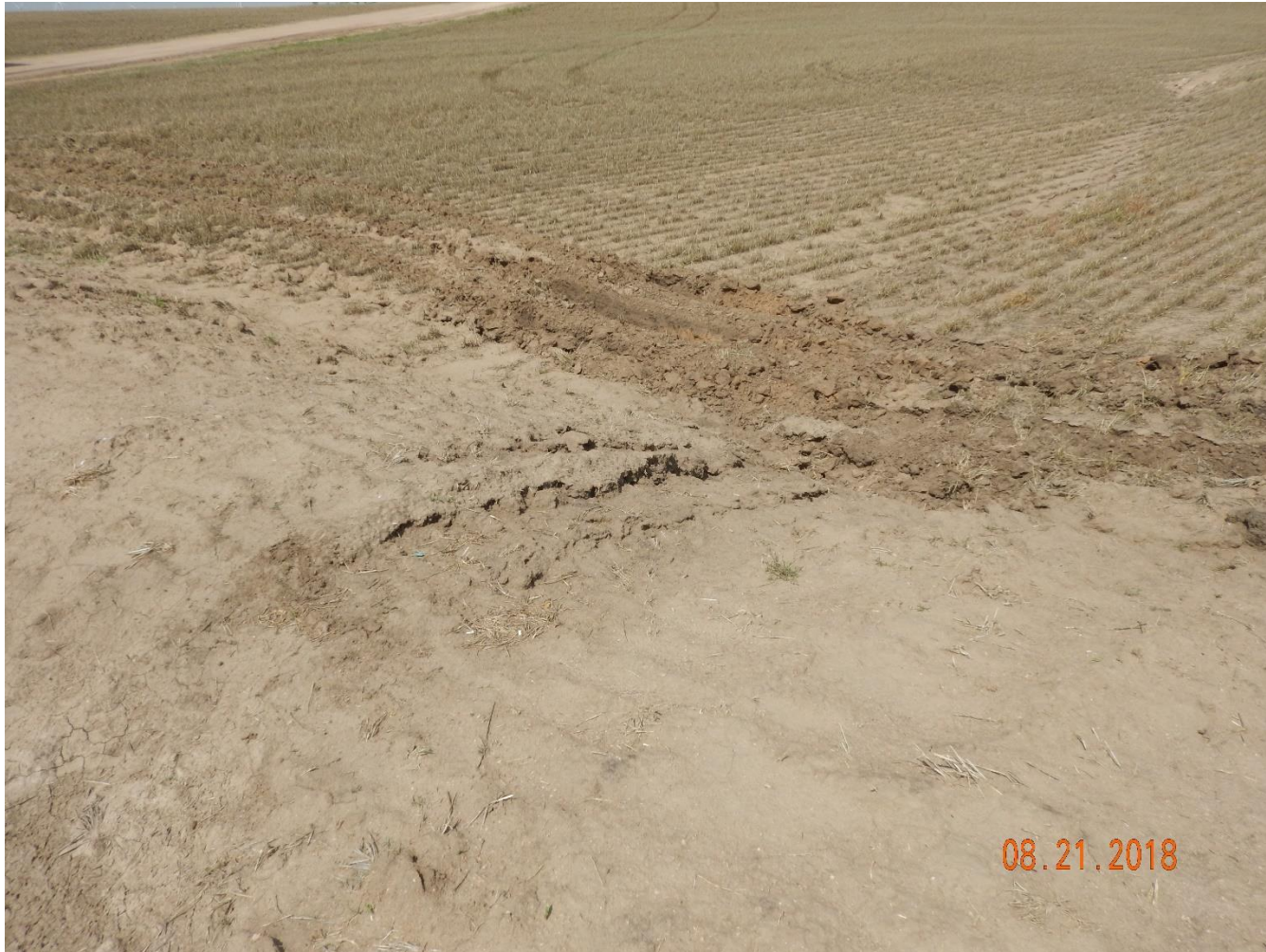
Photo 9: Continued from photo 8. Photo shows trap/pond does not have sufficient inlet or outlet protection in accordance with good engineering practice.
