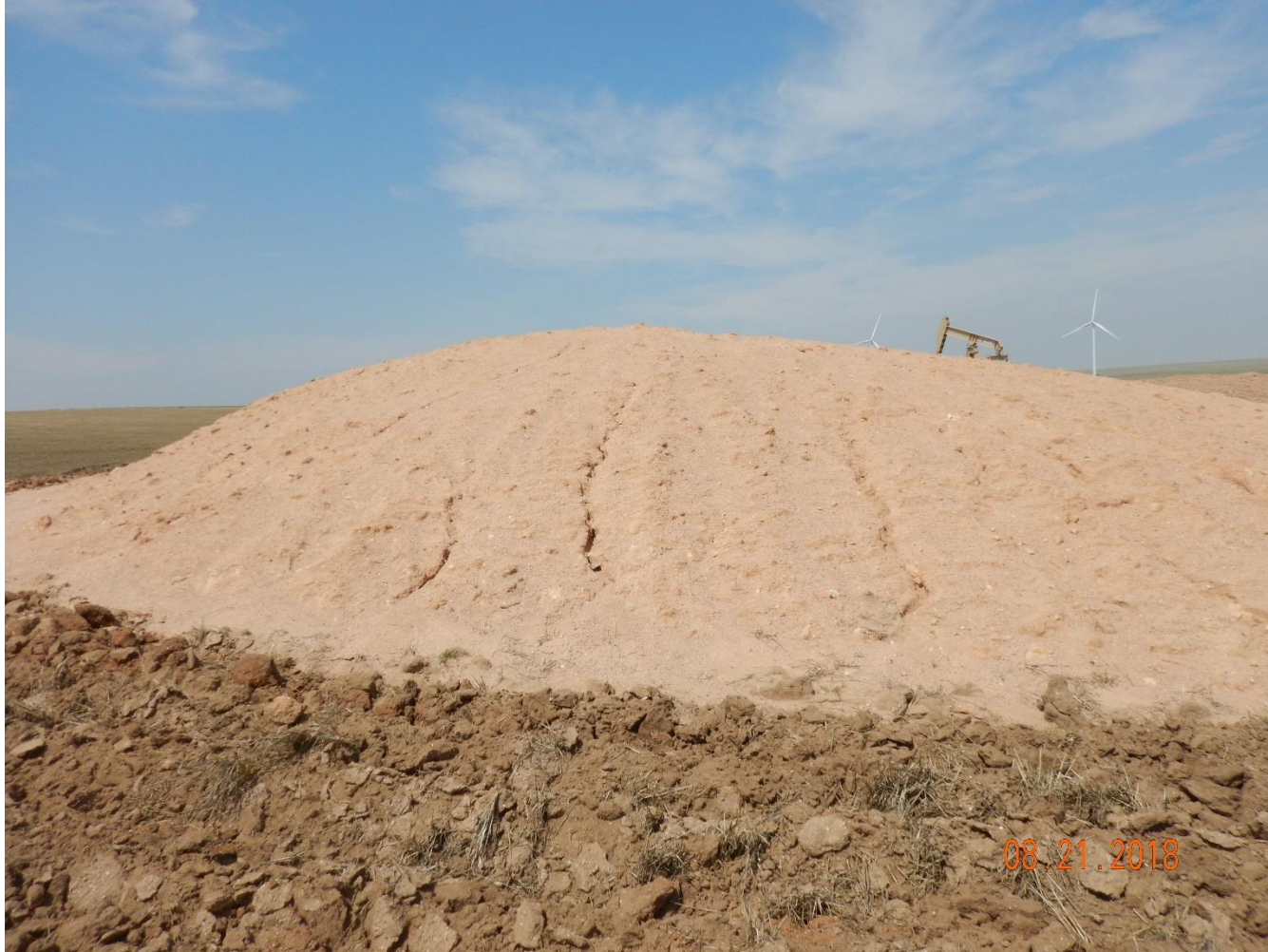
Photo 15: Photo taken from the southeast corner of the location, facing northwest. Photo shows sub-soil stockpile on locaiton. Erosion degradation evident on stockpile.
