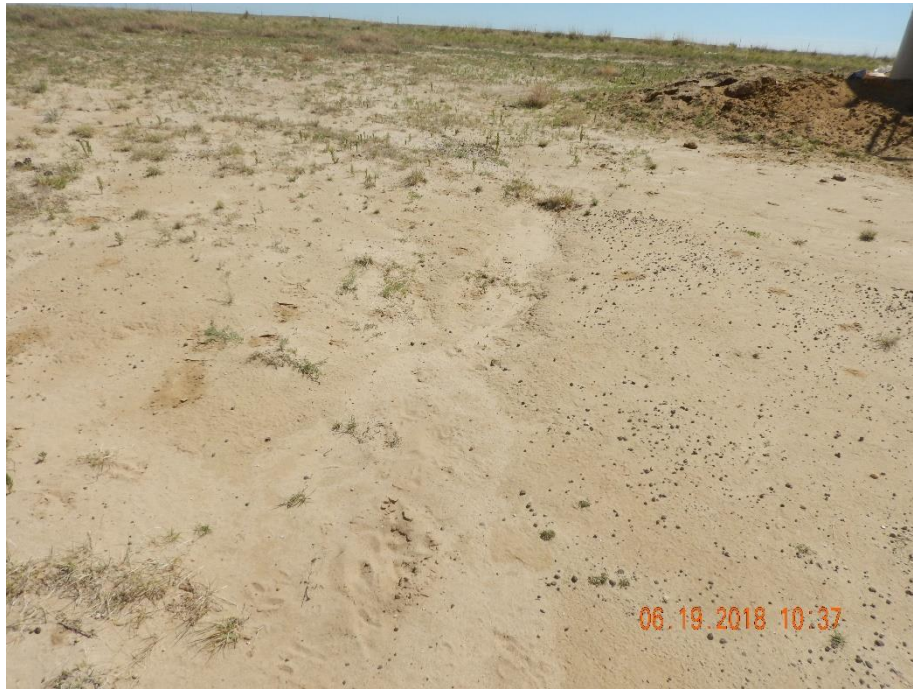
Photo 23: Photo taken from the northwest corner of the tank battery, facing east. Photo shows erosion degradation. Stormwater appears to be running off from the area of the tank battery, traveling downhill towards the location.
