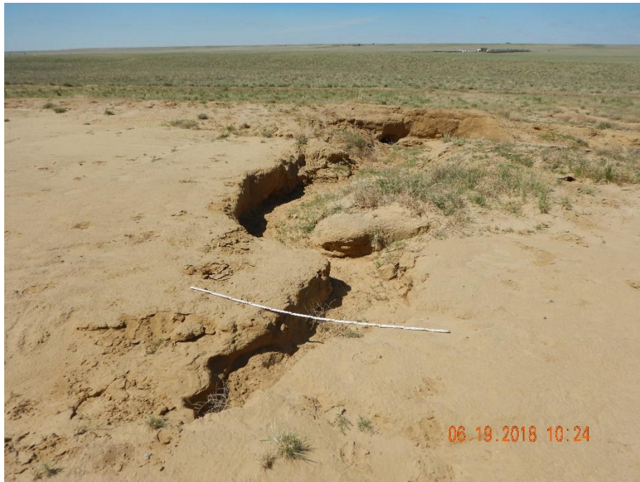
Photo 7: Photo taken from the large gully on northwest end of the production area, facing west. Photo shows erosion degradation has continued to expand and degrade both the production and interim area. 6 foot measuring stick for reference
