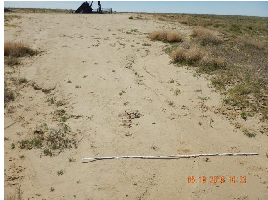
Photo 2: Photo taken from the access road on the north end of the location, facing north. Photo shows stormwater erosion has continued to degrade the location. 6 foot measuring stick for reference.
