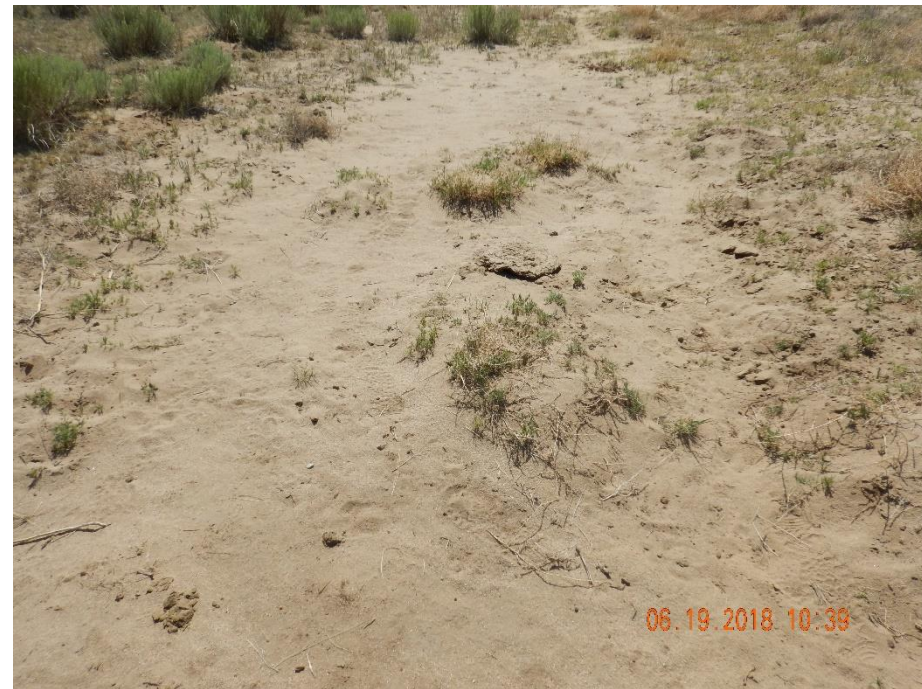
Photo 30: Photo taken from the access road. Photo shows pedestal formations due to stormwater degradation. Pedestals form when stormwater erodes away un-stabilized areas of soil around vegetation.
