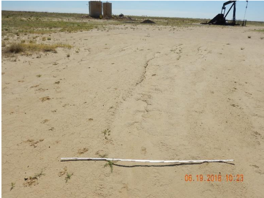
Photo 3: Photo taken from the access road on the north end of the location, facing north. Photo shows stormwater erosion has continued to degrade the location. 6 foot measuring stick fore reference.
