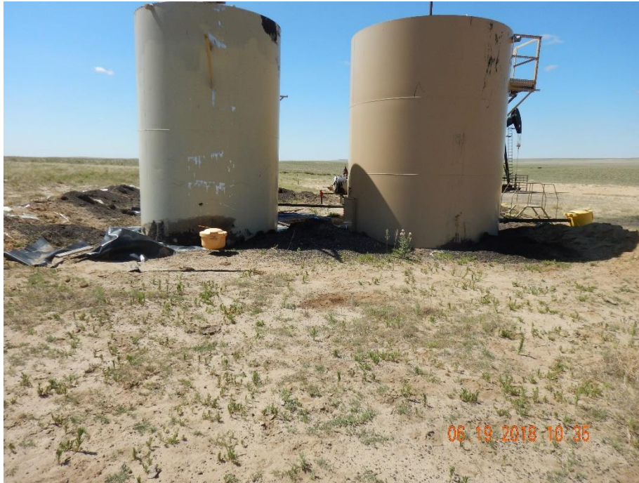
Photo 21: Photo taken from the north end of the tanks on location, facing south. Previous photos documented that the berms around the tanks were inadequate and required operator to repair or install berms, or other secondary containment devices. Photo shows berms, or other secondary containment devices have not been repaired or installed. Photo also shows incomplete signage on tanks, including NFPA diamond labeling.
