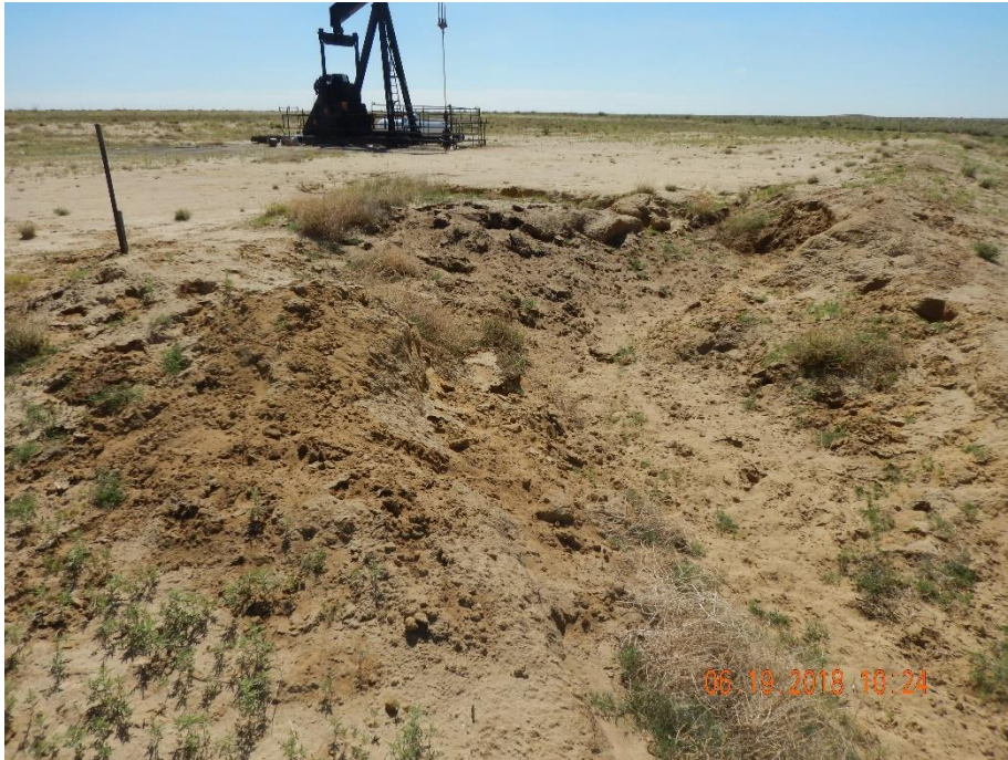
Photo 5: Photo taken from the northwest end of the production area, facing south. Photo shows stormwater erosion has continued to degrade the location. The large gully has continued to expand. 6 foot measuring stick fore reference.
