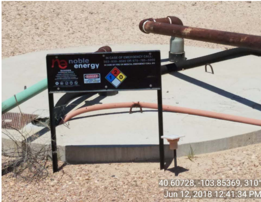
Photo 4: No capacity at produced water vault
