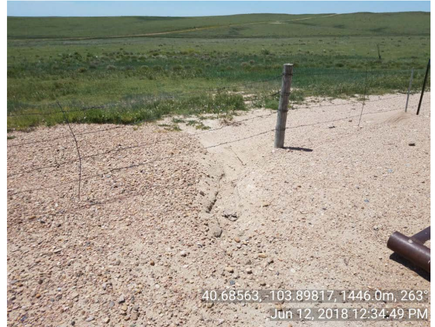
Photo 3: Stormwater erosion S of wellhead
