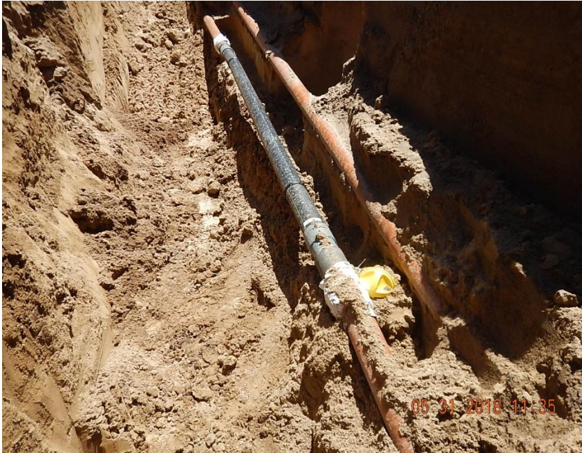
View of follow-up repair completed to the damaged section of flowline; HDPE pipe section replaces damaged section of flowline. GPS marker ball placed in area of repair
