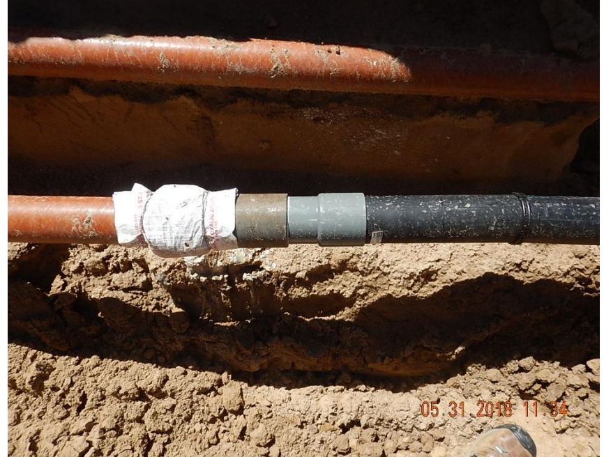
Closer view of the transition between existing fiberglass flowline and replacement section of (HDPE/ Poly) pipe
