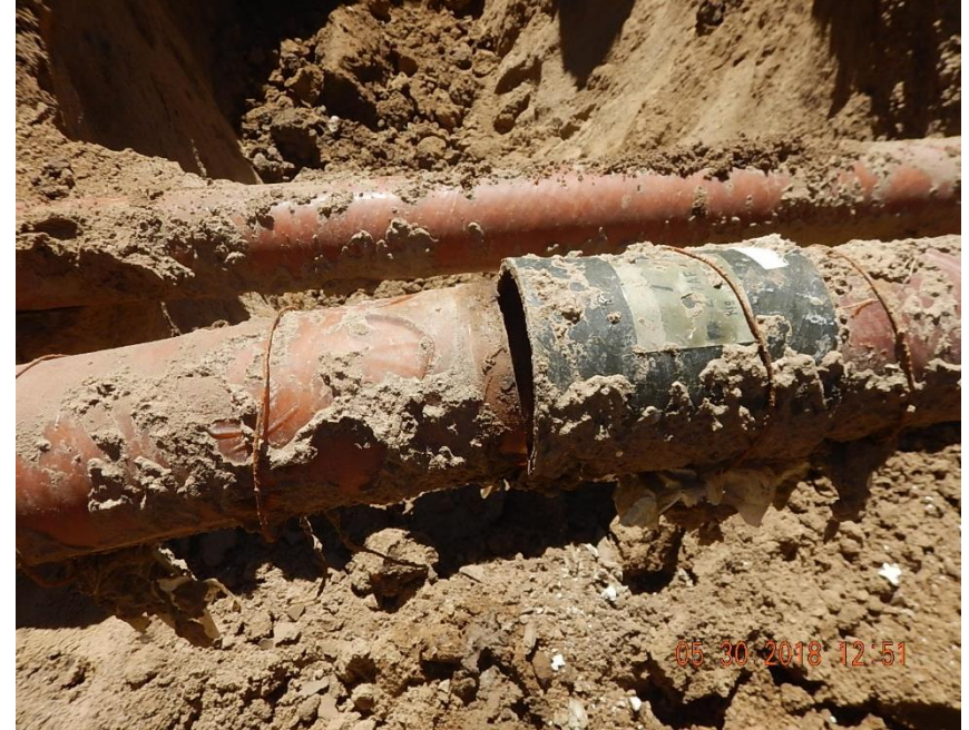
Photo of failed repair completed by contractor (no longer working on this project); Fiberglass coupler improperly installed, no adhesive used to complete connection
