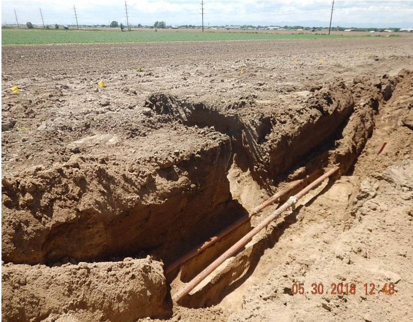
Photo taken 5/30/18 of excavation exposing (2) Hyndrex Resources 3" fiberglass flowlines; initial (failed) repair can be seen on Northern most flowline
