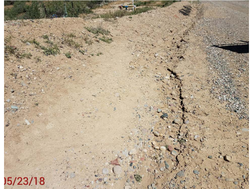
Location Photo #6, Erosion along West side of access road
