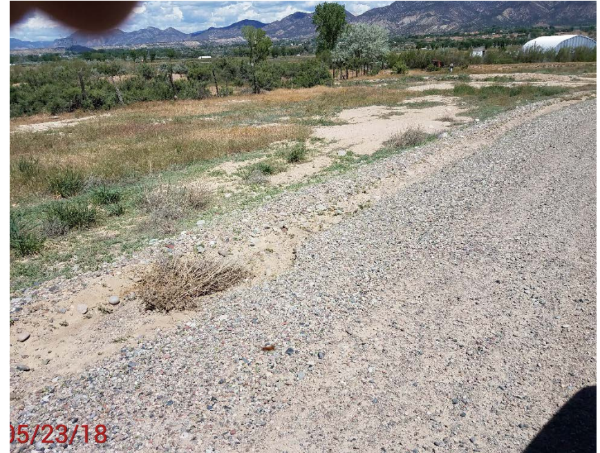
Location Photo #8, Erosion along West side of access road
