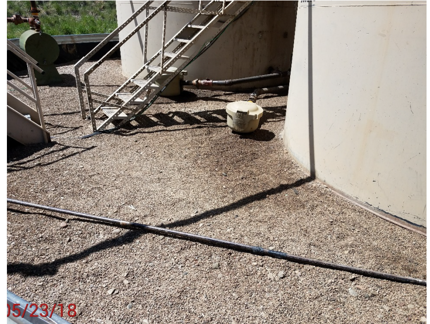
Location Photo #2, Stained material in tank containment
