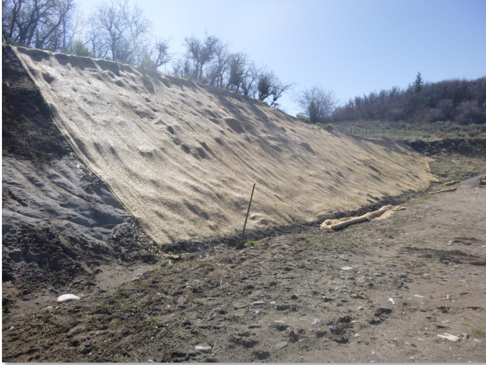
Photo 1. Installation of Jute matting in process 4/30/2018.
