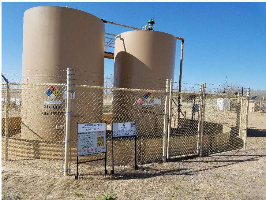
Photo 3. Tank battery
