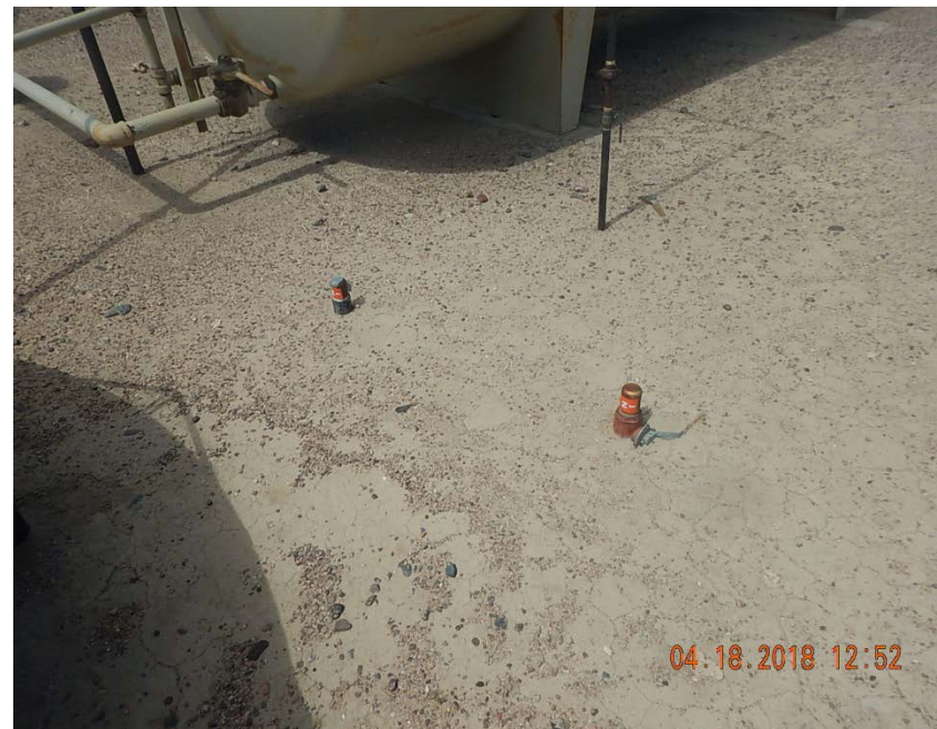
Photo 8: Marked, plugged risers at tank.
