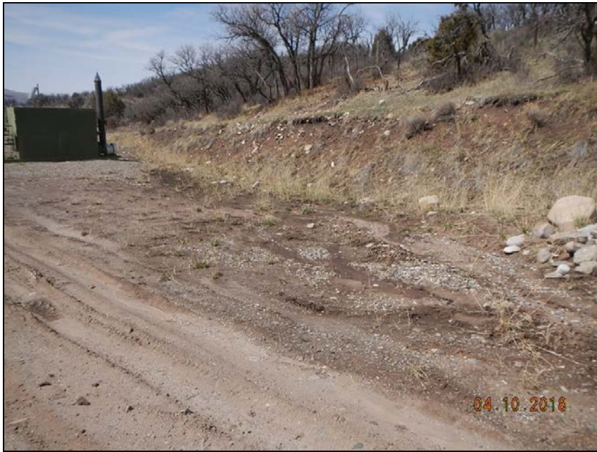
Photo 1. Erosion and sediment migration on to location.
