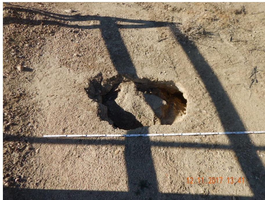
Photo 6: Photo dated 12/11/2017. Photo shows subsidence has not been repaired, and has been allowed to continue to expand. 6 foot measuring stick for reference.
