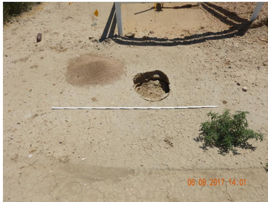
Photo 4: Photo from previous inspection dated 6/8/2017. Previous inspections required operator to repair subsidence concerns occurring on the former battery location. Photos 4-6 date from 6/8/2017 to 12/11/2017 show subsidence has not been repaired and degradation has continued, and hole has expanded. 6 foot measuring stick for reference.
