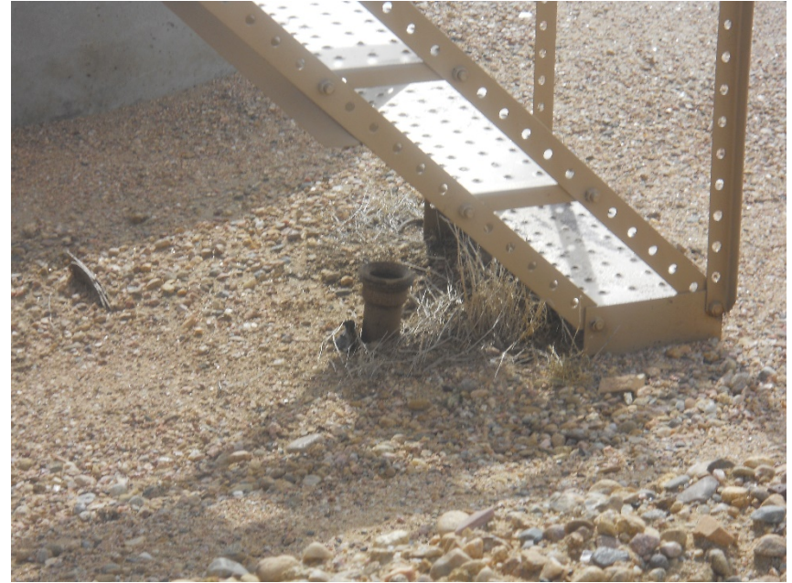
2" unused/unmarked steel riser under the stairs to the crude oil tank
