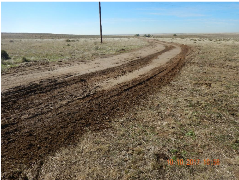
Photo 2: Photo taken from the access road, north of the location. Photo shows portion of the North/South access road requiring reclamation. The contractor on site had stated topsoil had been brought in to fill the road.
