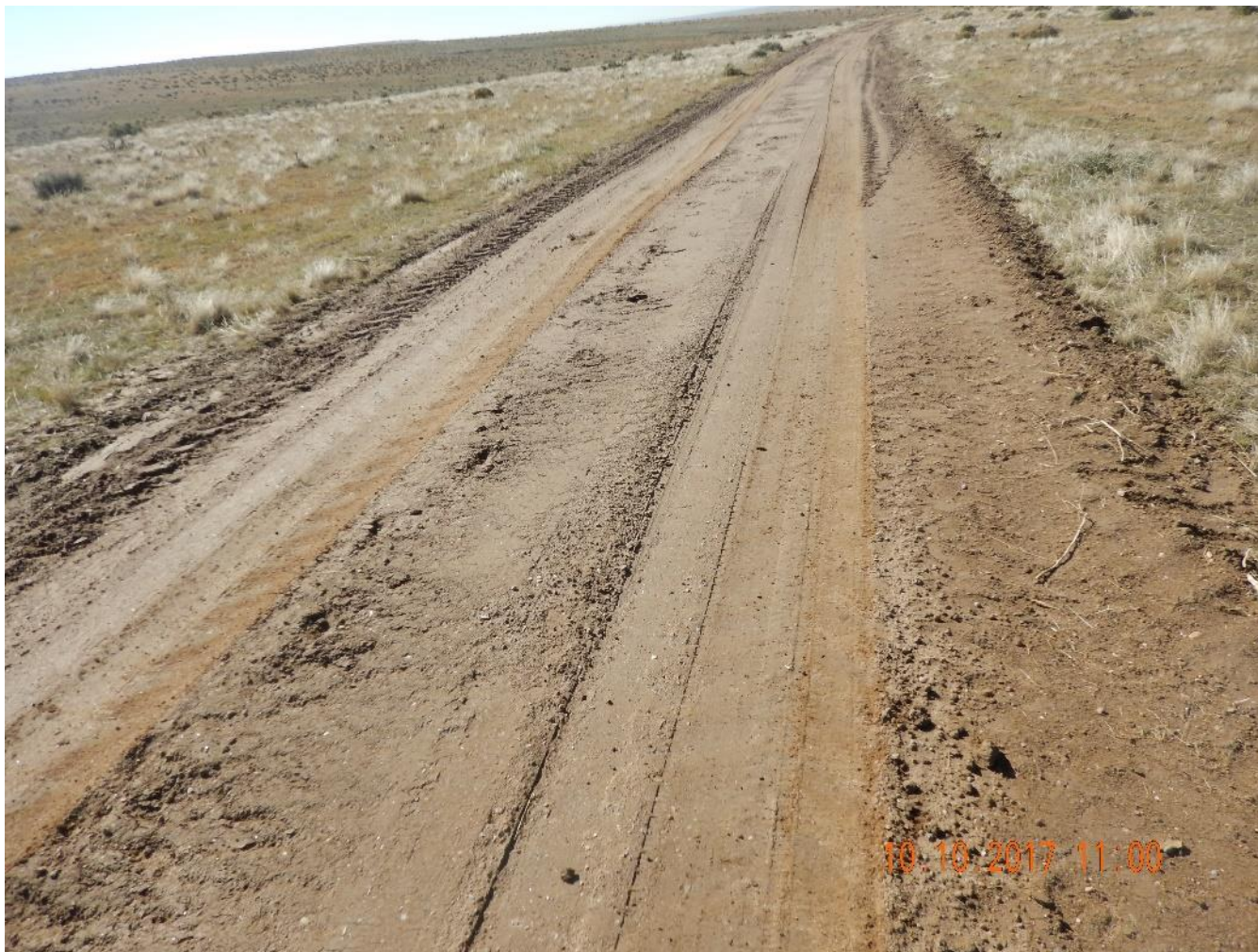
Photo 4: Photo taken from the access road, north of the location. Photo shows topsoil had been brought in for the road. Note: COGCC reclamation rules require access roads to be cross ripped to a depth of 18 inches. After conversations with the contractor on site at time of inspection, it was indicated that the required compaction alleviation had not yet been conducted, and that there was no schedule to perform the work.
