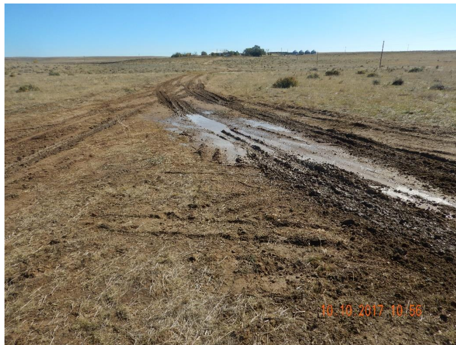
Photo 3: Photo taken from the access road, north of the location. Photo shows portion of the East/west portion of the road not being reclaimed. The contractor on site had stated that any gravel or road base removed from the access road, had been placed on this section of the road for the surface owner.
