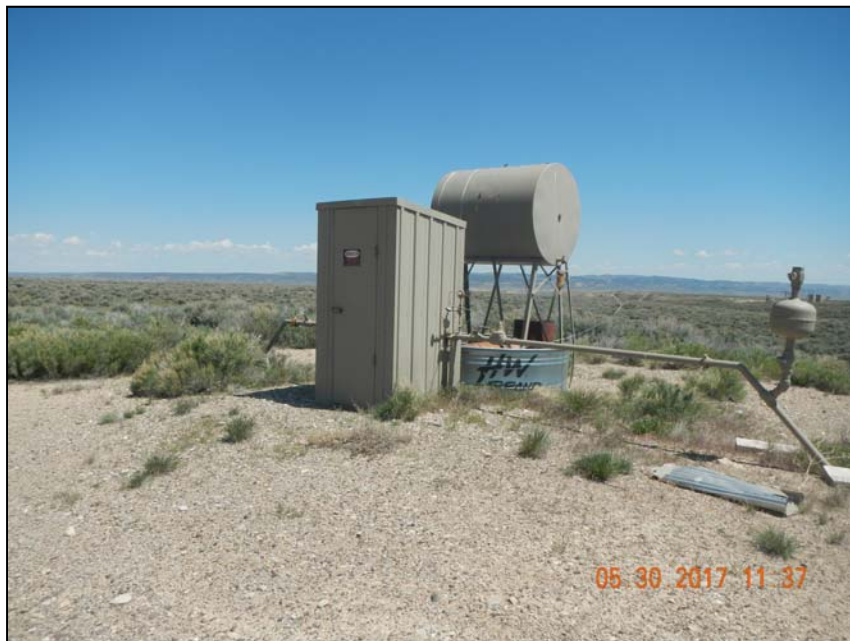
Photo 6. 2 – 2" steel risers at meter run. Unlabeled container in background.
