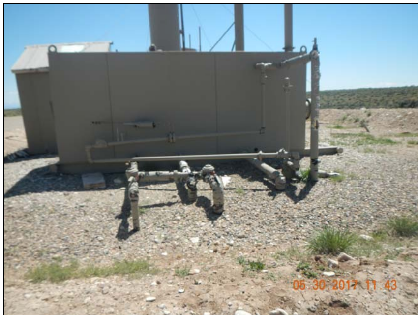
Photo 10. Risers at horizontal separator.
