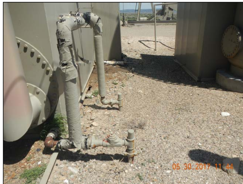
Photo 11. Risers at vertical separator on right and horizontal separator on left.
