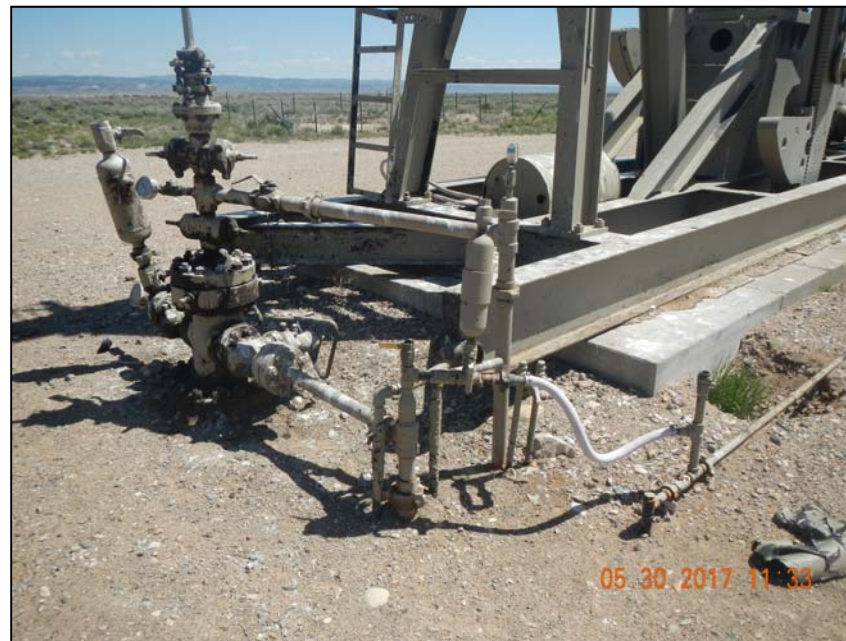
Photo 3. 2 – 2" steel riser, 2 – 1" insulated steel riser, 3 – 1" steel riser at wellhead
