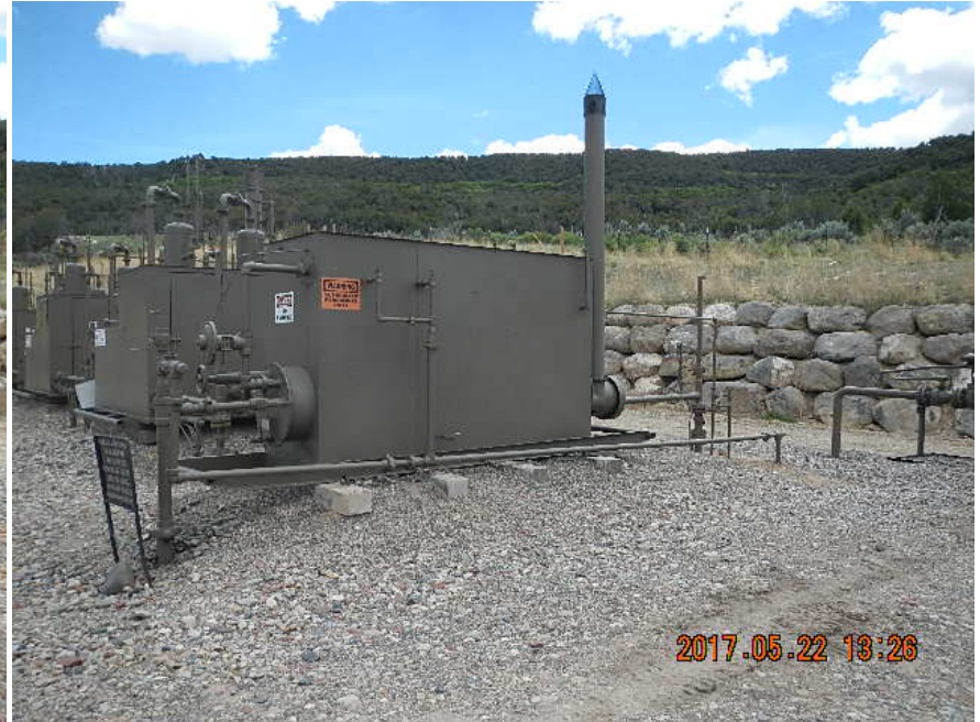
Single horizontal heated separator with 1-3" steel input from well; 1-2" steel water/oil line out to tank battery; 1-3" steel gas line out to sales meter; 2-1" steel risers out.
