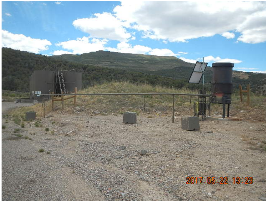
Emission device – 2- 3” steel lines, one not in use. 1 -1” gas supply line
