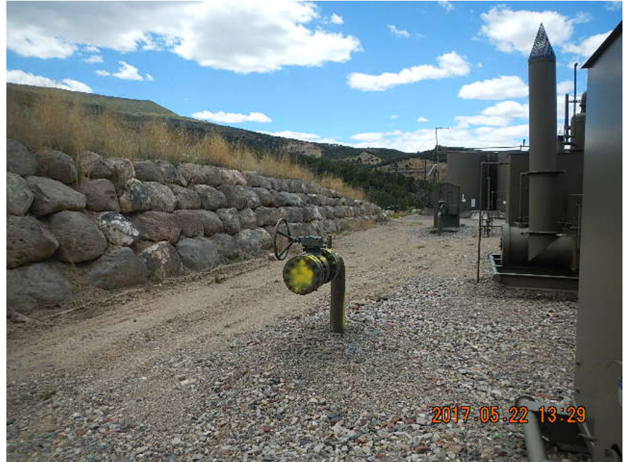
6" steel riser with gate valve and blind flange – ties into midstream
