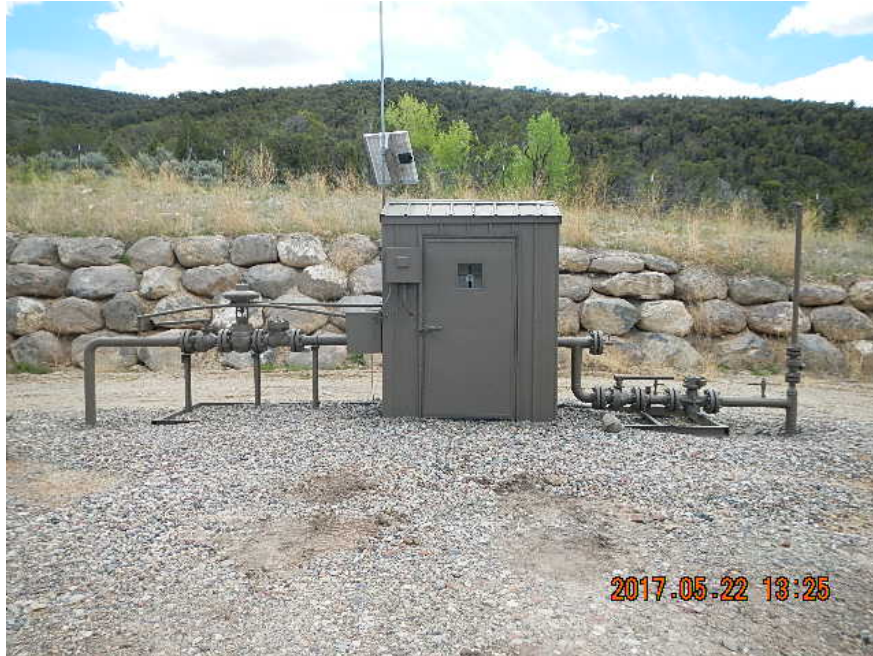
Gas meter with 2-4" steel risers at gas meter
