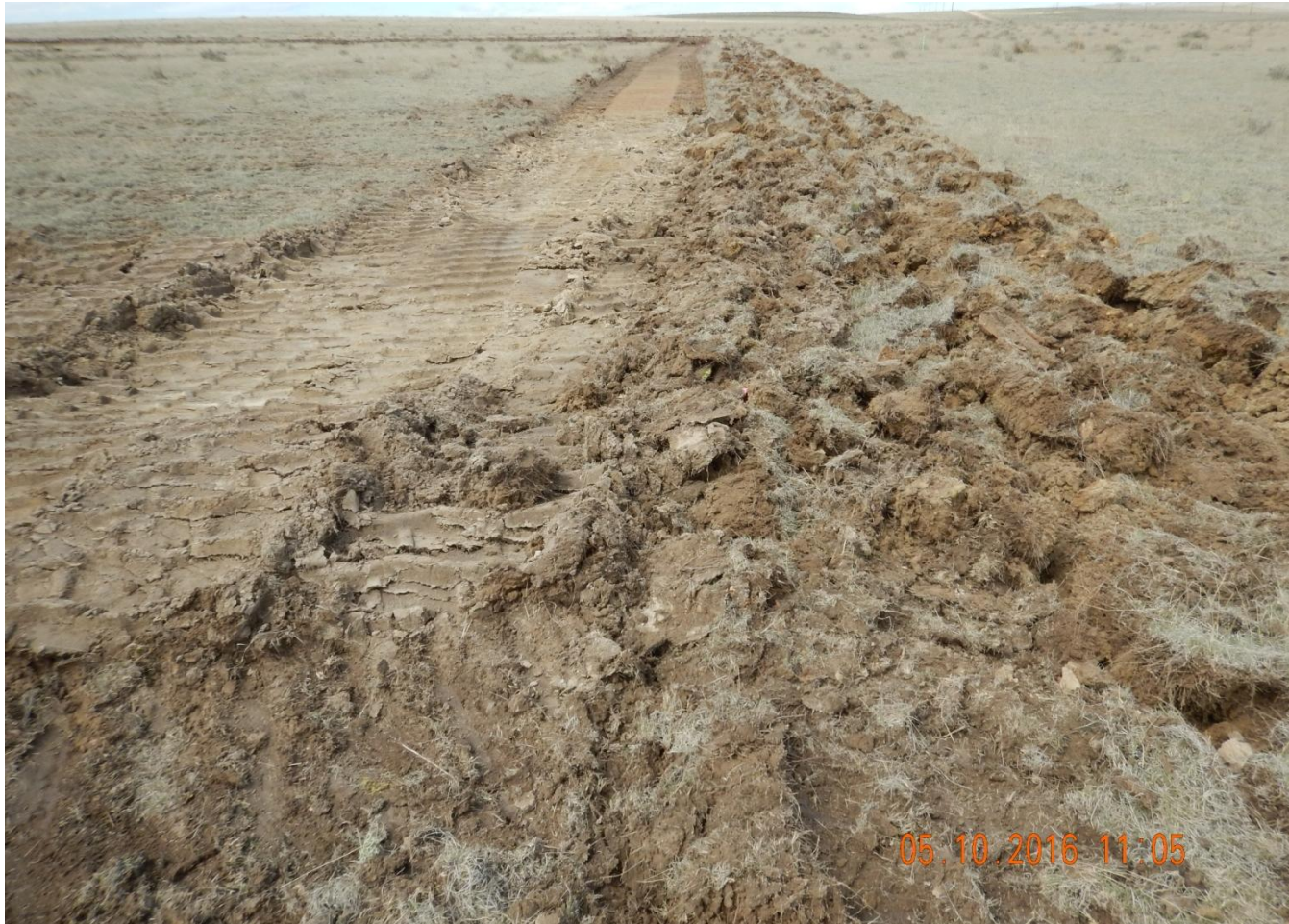
Photo 1. Photo taken from northeast location, facing West. Temporary BMP installed in center of photo while topsoil salvage is in process. Permanent BMPs will be installed upon completion of topsoil salvage.
