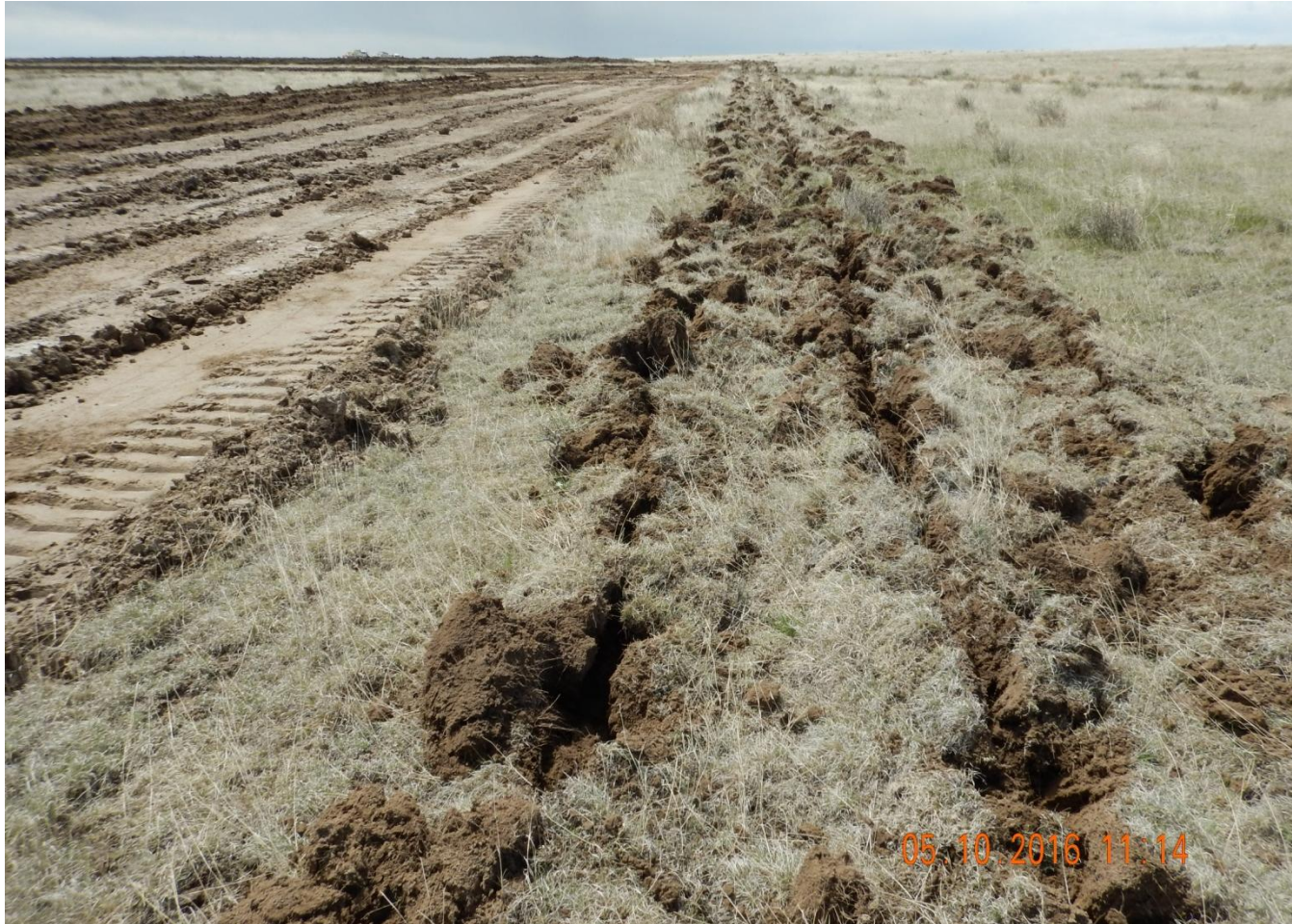
Photo 3. Photo taken from northwest location, facing South. Temporary BMP installed in center of photo while topsoil salvage is in process. Permanent BMPs will be installed upon completion of topsoil salvage.
