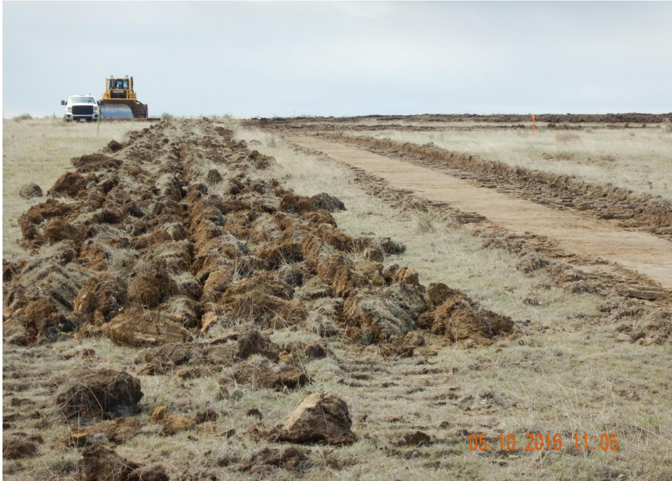
Photo 2. Photo taken from northeast location, facing South. Temporary BMP installed in center of photo while topsoil salvage is in process. Permanent BMPs will be installed upon completion of topsoil salvage.
