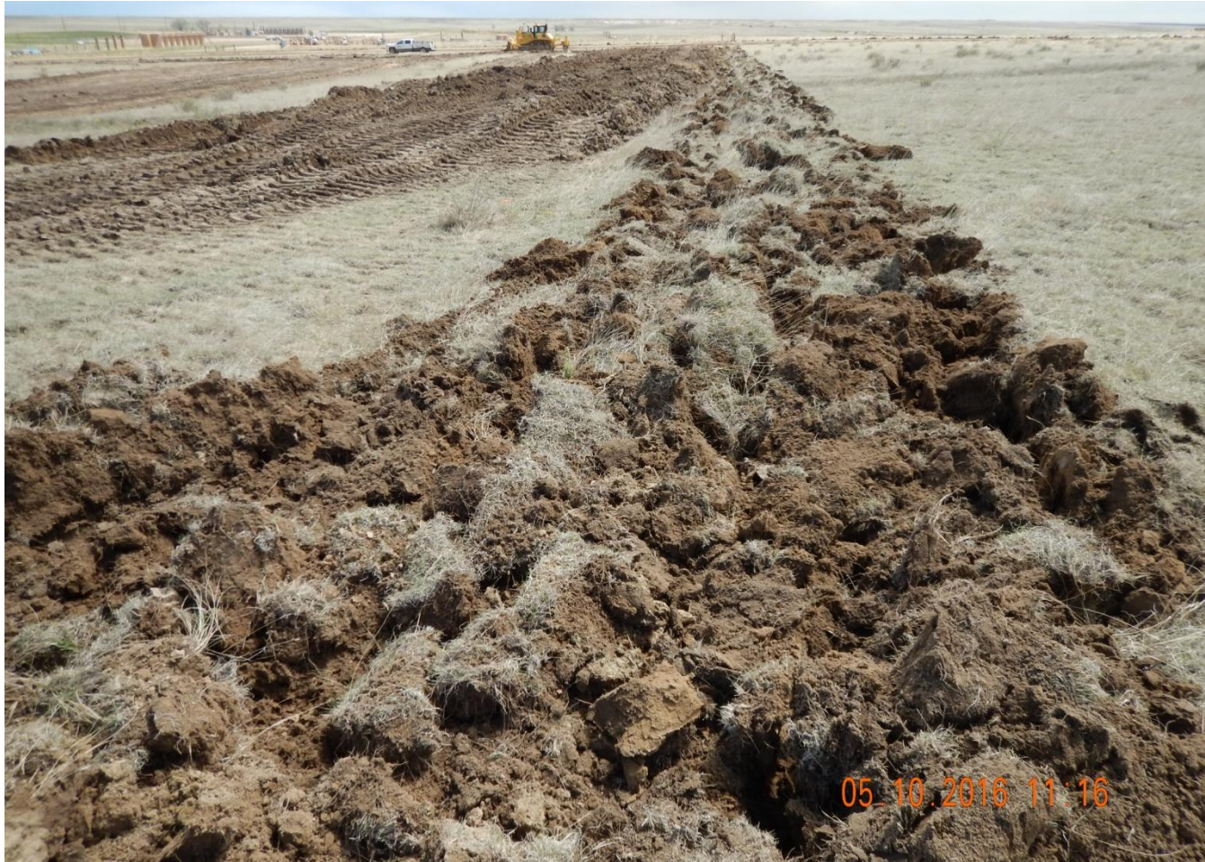
Photo 4. Photo taken from southwest location, facing East. Temporary BMP installed in center of photo while topsoil salvage is in process. Permanent BMPs will be installed upon completion of topsoil salvage.
