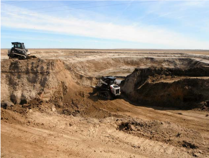
Rebuilding of wall between pits after excavation
