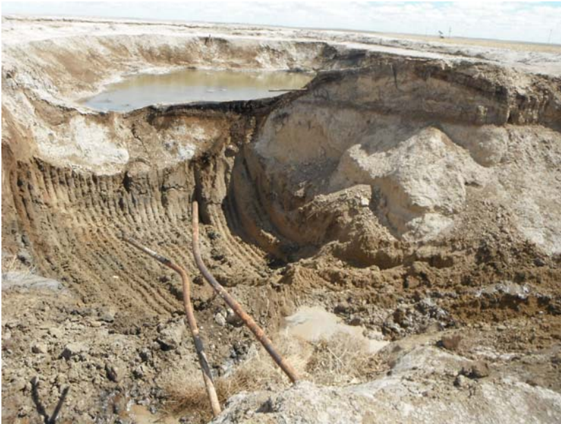
Collapsed wall between evaporation pit and skim pit
