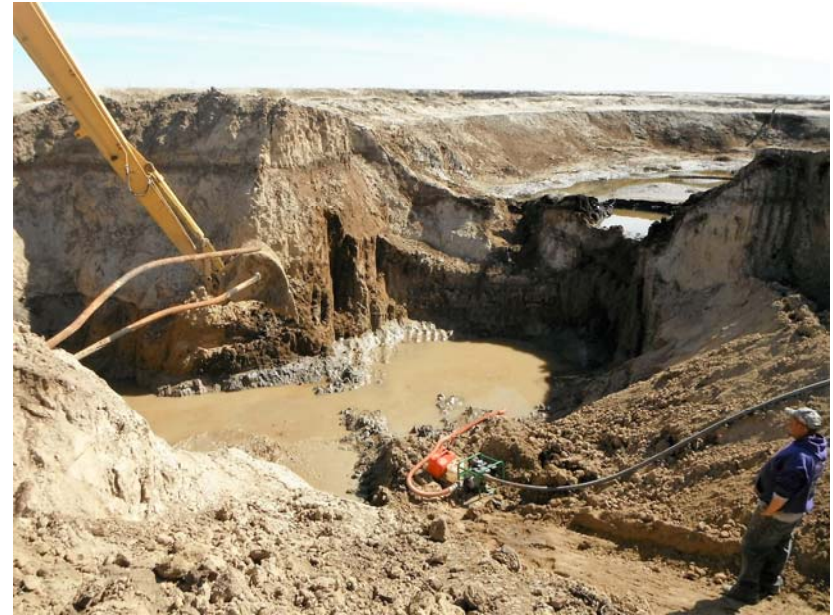
Dewatering of skim pit excavation
