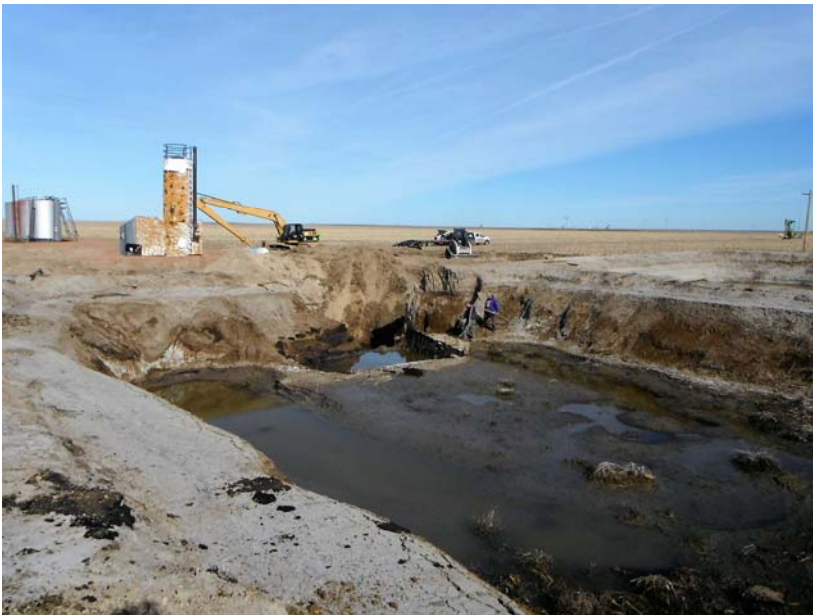
Collapsed wall from evaporation pit side
