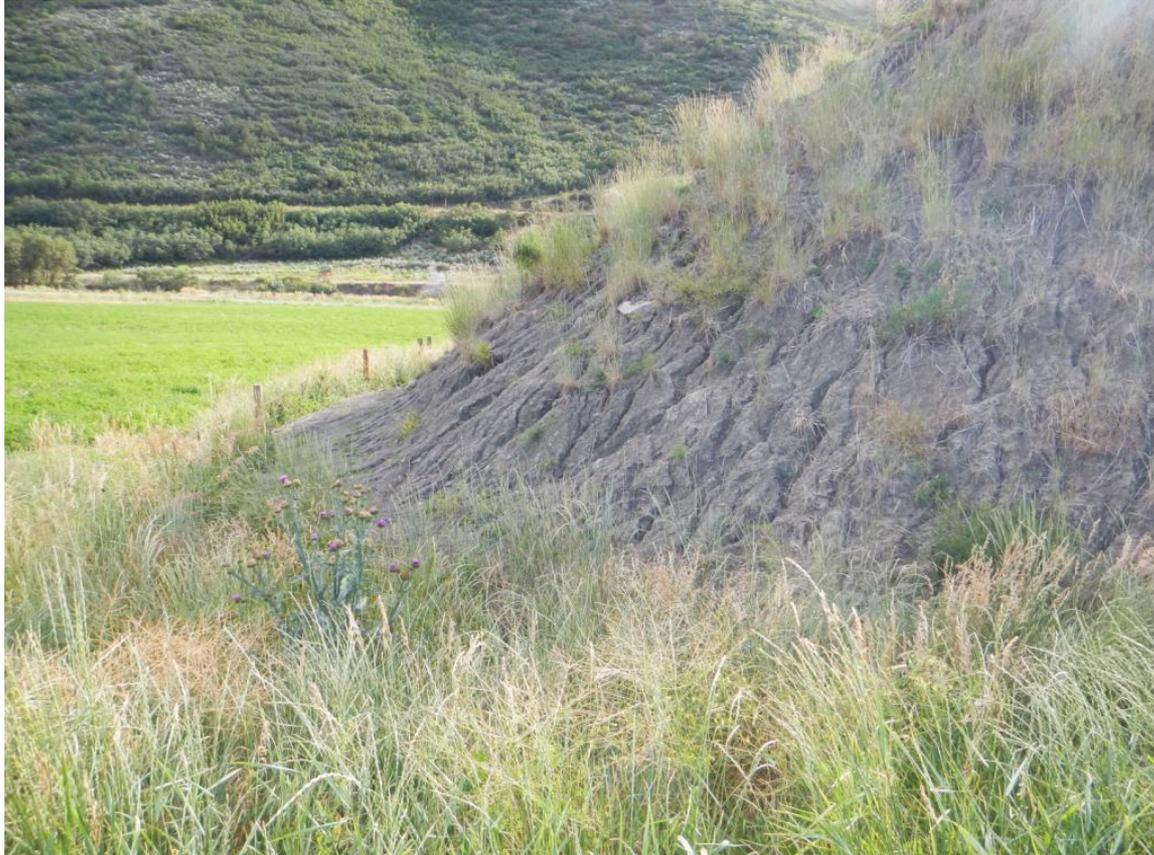
Photo 5: Rill erosion on fill slope
