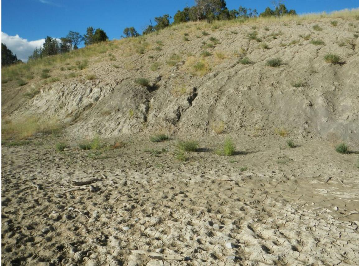
Photo 3: Cut slope rill and gully erosion
