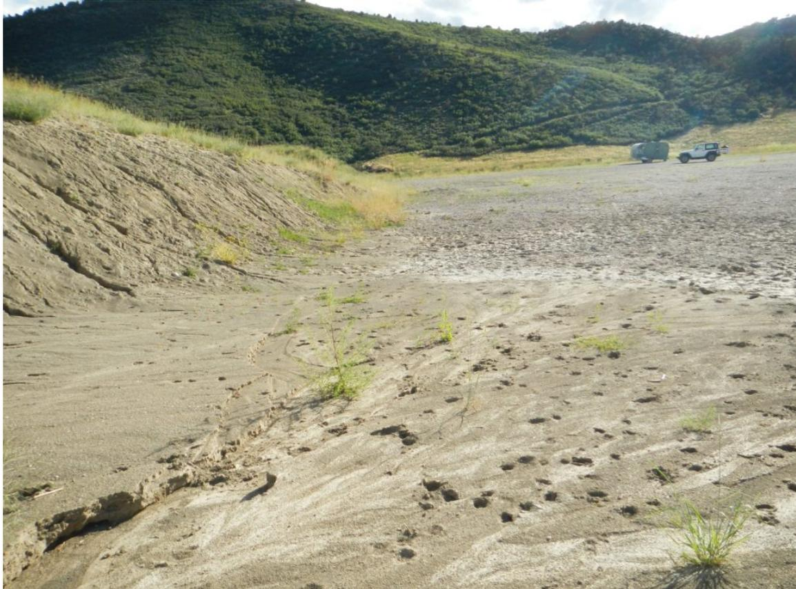
Photo 4: Run on from Cut slope rill and gully erosion.
