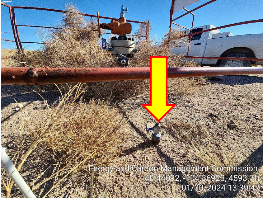
Photo 3 – Unmarked Riser
