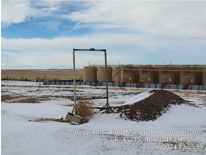
Photo 3 – Automation Stand at Wellsite
