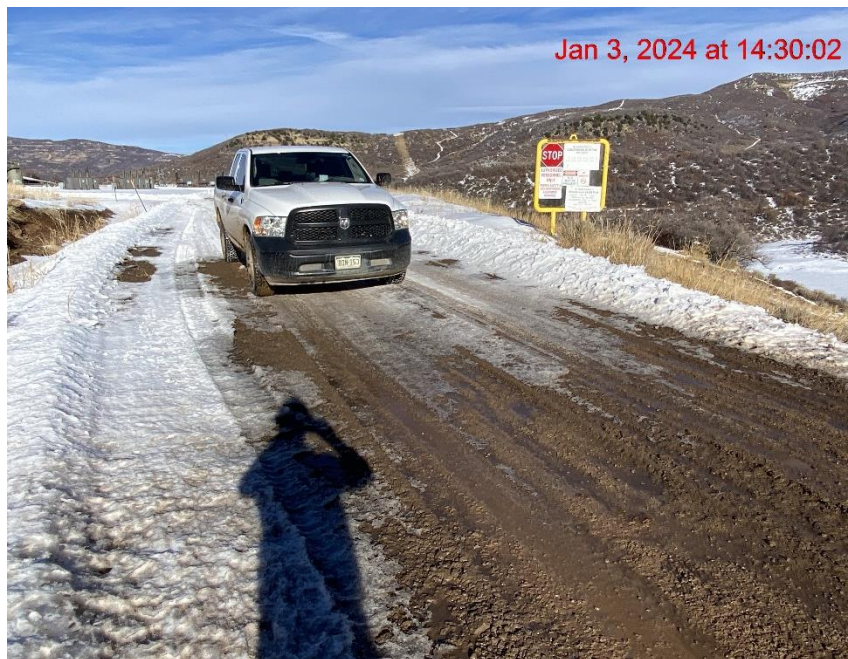
Insufficient Vehicle Tracking BMPs at Location Entrance/Exit – Photo #08481
