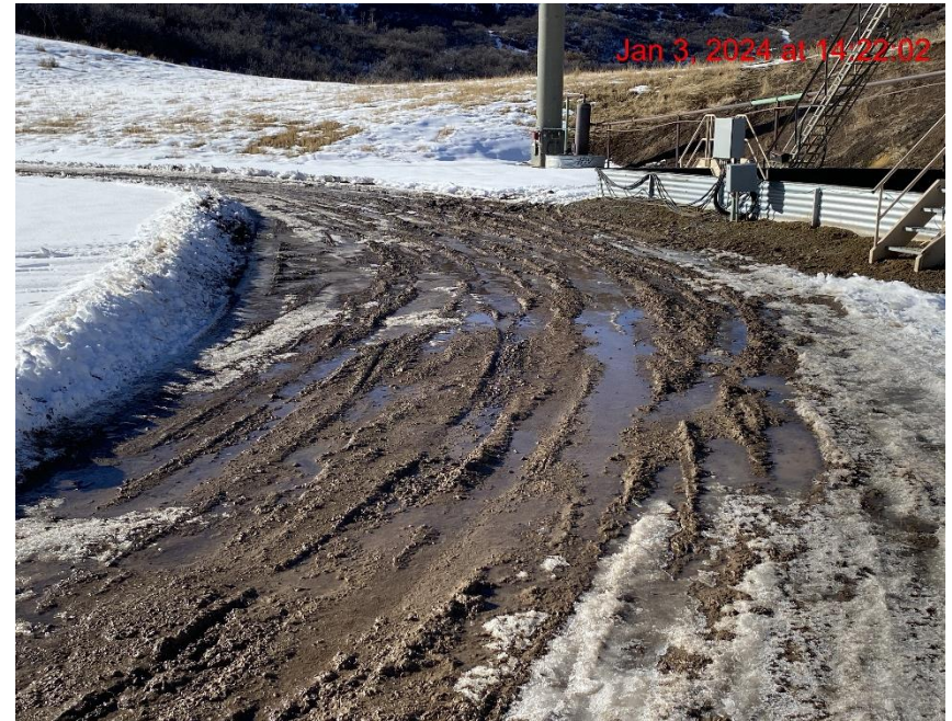
Lack of Stabilization – Photo #08473
