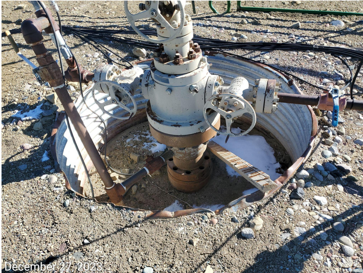
Photo 3: Photo example showing cellars at wells remain open. .
