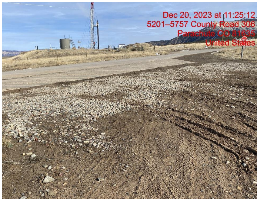
Insufficient Vehicle Tracking BMPs at Location Entrance/Exit – Photo #08323
