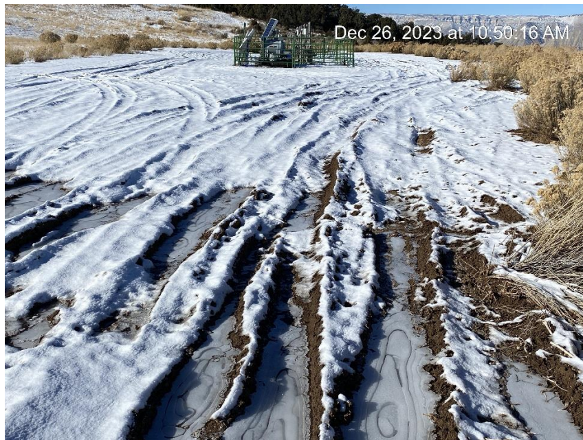
Lack of compaction accessing wellheads
