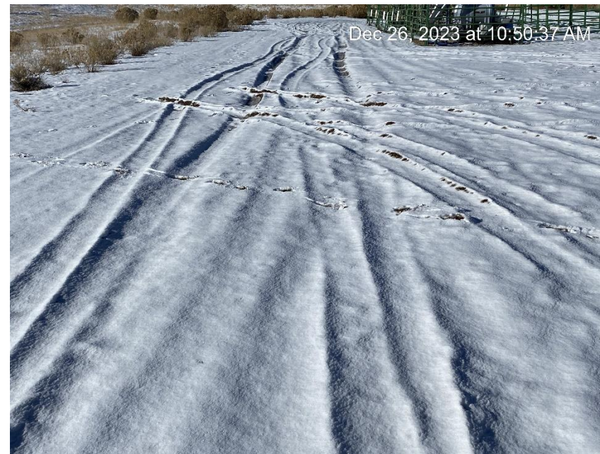
Lack of compaction around wellheads
