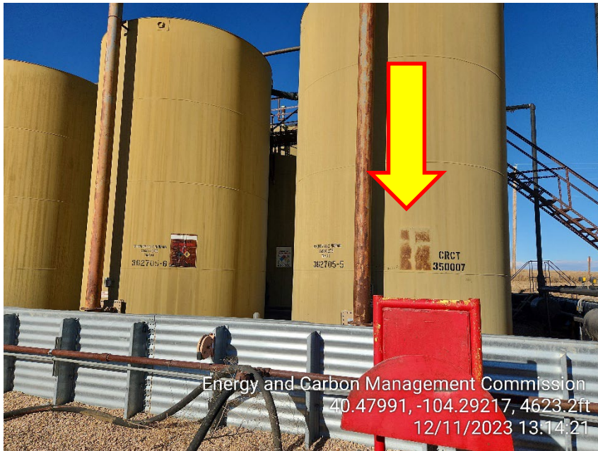
Photo 17 – NFPA, Content and Capacity Labels missing on SE Tank
