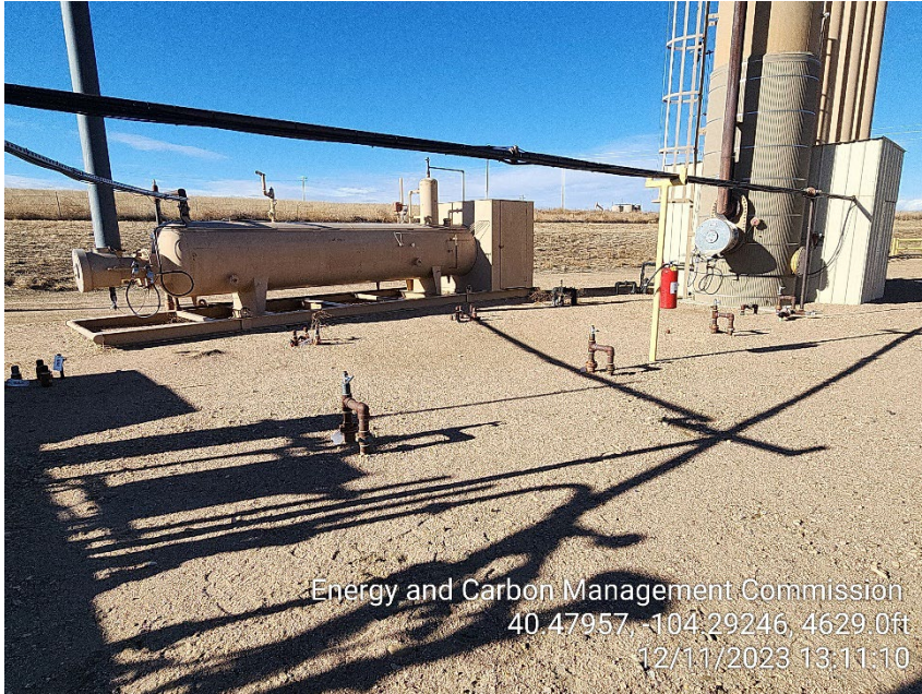
Photo 7 – Separator and Heater Treater
