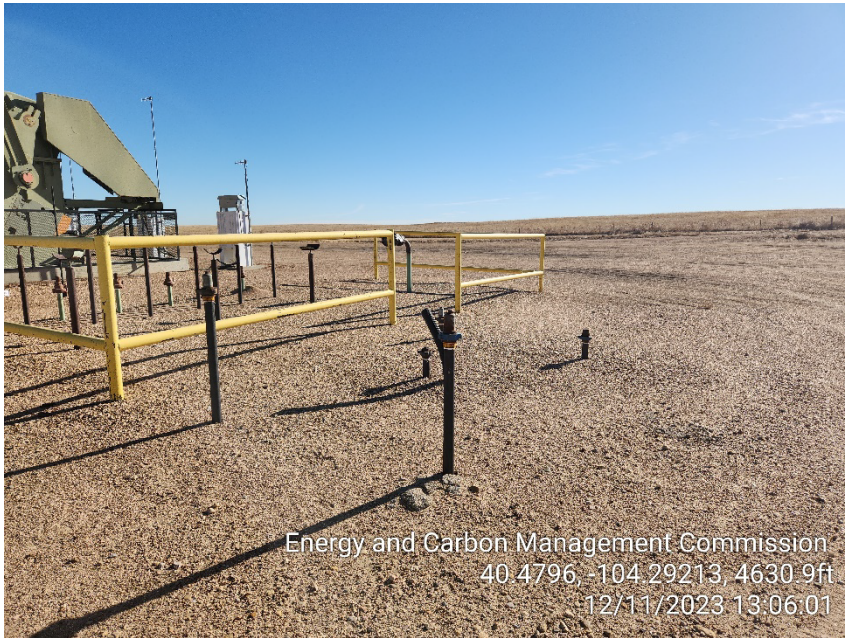
Photo 3 – 2” Riser West of Pumping Units not OOSLAT
