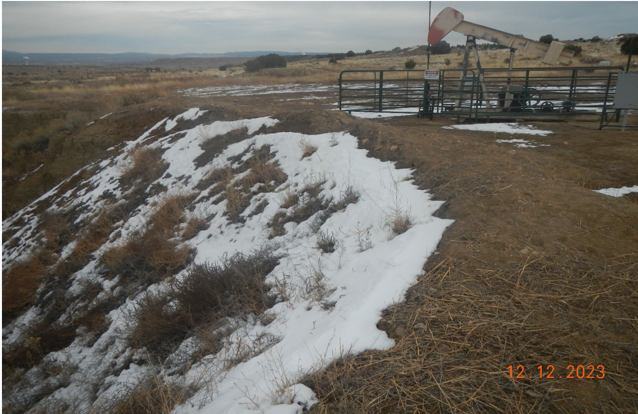
Photo 5. Facing toward the embankment. This area needs to be seeded for stabilization of the embankment or other BMP may be utilized. Shrubs in the area that are easily established include Rubber rabbitbrush and Four wing salt brush.
