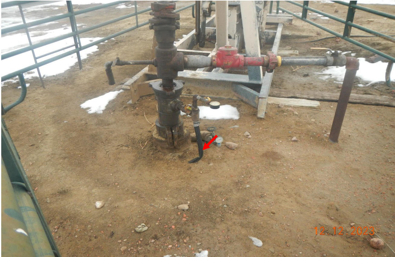
Photo 6. There is a black plastic pipe that is bent and an audible leak was heard from this area.
