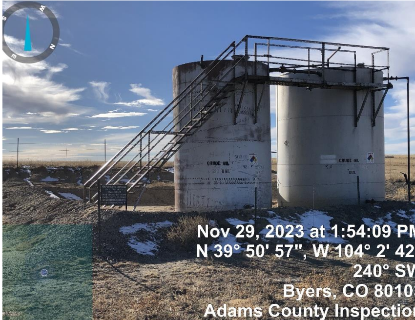
Photo#7 Production Tank and Produced Water Tank
