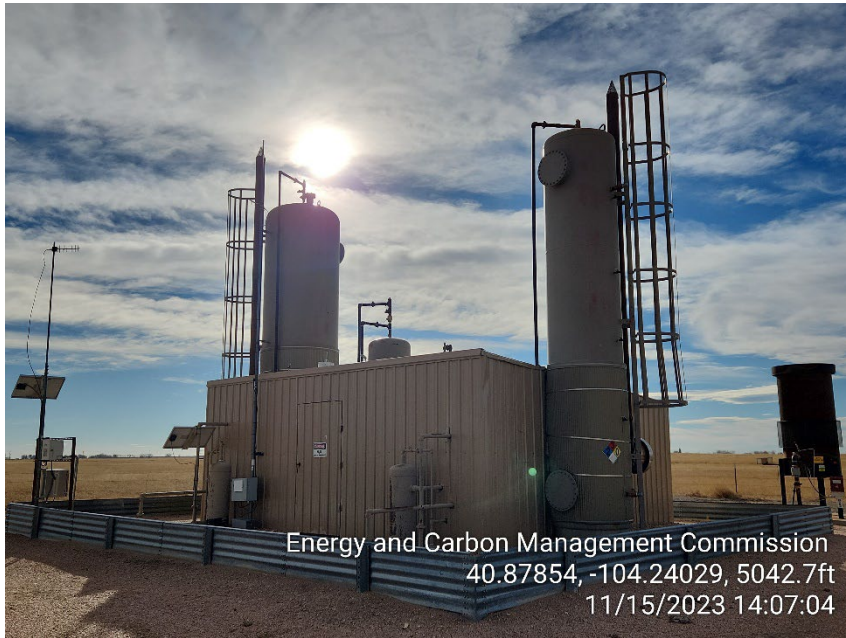
Photo 3 – Heater Treaters and ECD
