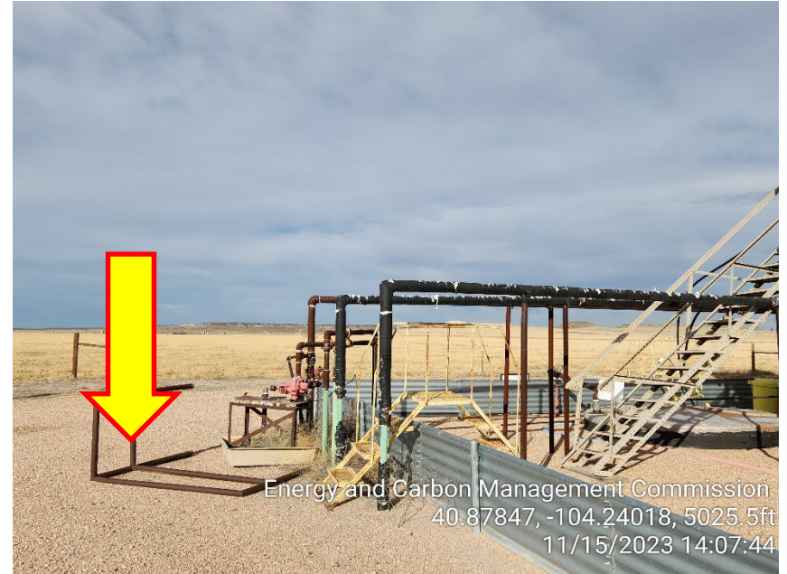
Photo 4 – Recycle Pump in disrepair
