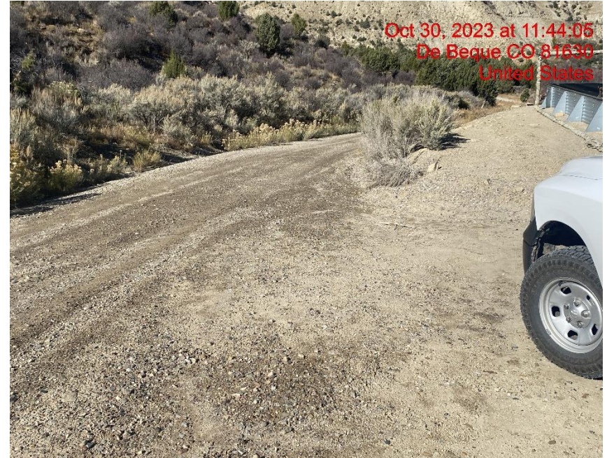
Insufficient Vehicle Tracking BMPs at Location Entrance/Exit – Photo #07231
