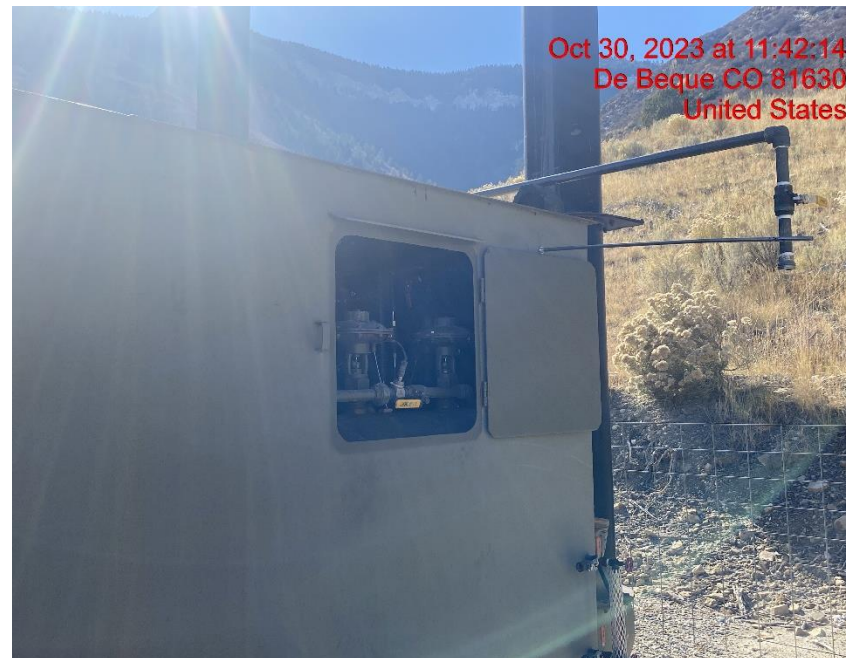
Unsecured Hatch on Separator – Photo #07226
