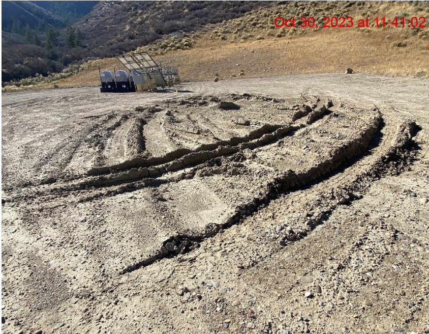
Lack of Stabilization – Photo #07224
