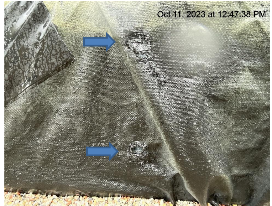
Photo # 2485 Holes in containment liner/liner needs maintenance
