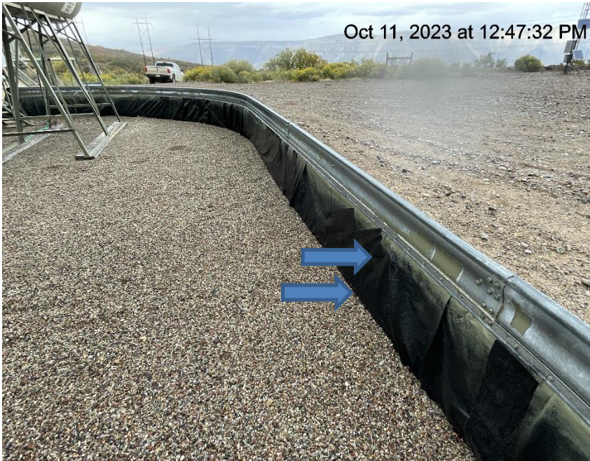
Photo # 2484 Holes in containment liner/liner needs maintenance
