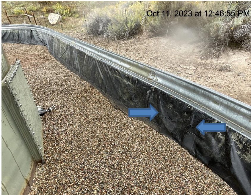
Photo # 2482 Holes in containment liner/liner needs maintenance
