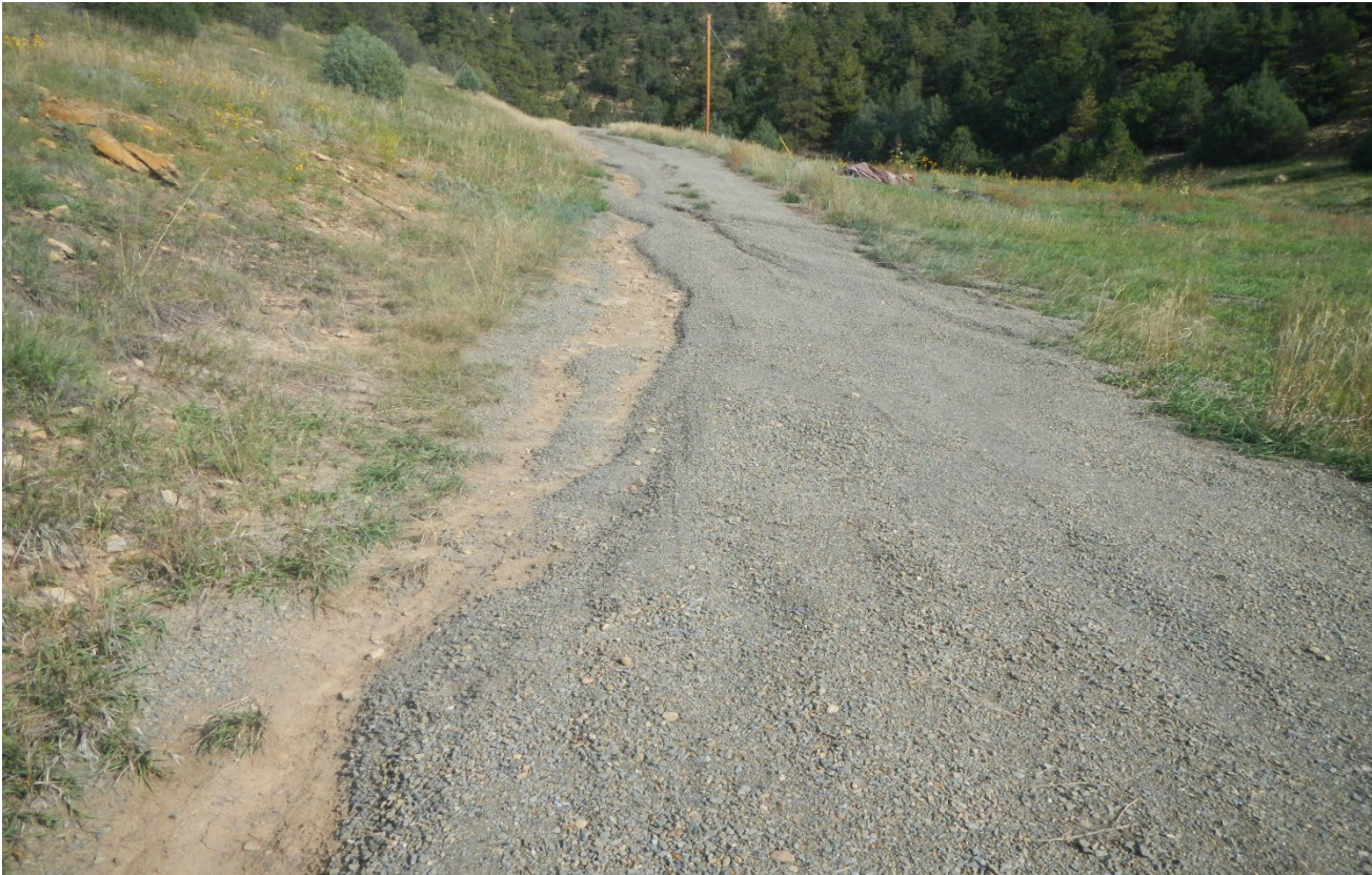
Photo 1. Facing north at the beginning of the access road. Stormwater run-on has caused erosion along the road.
