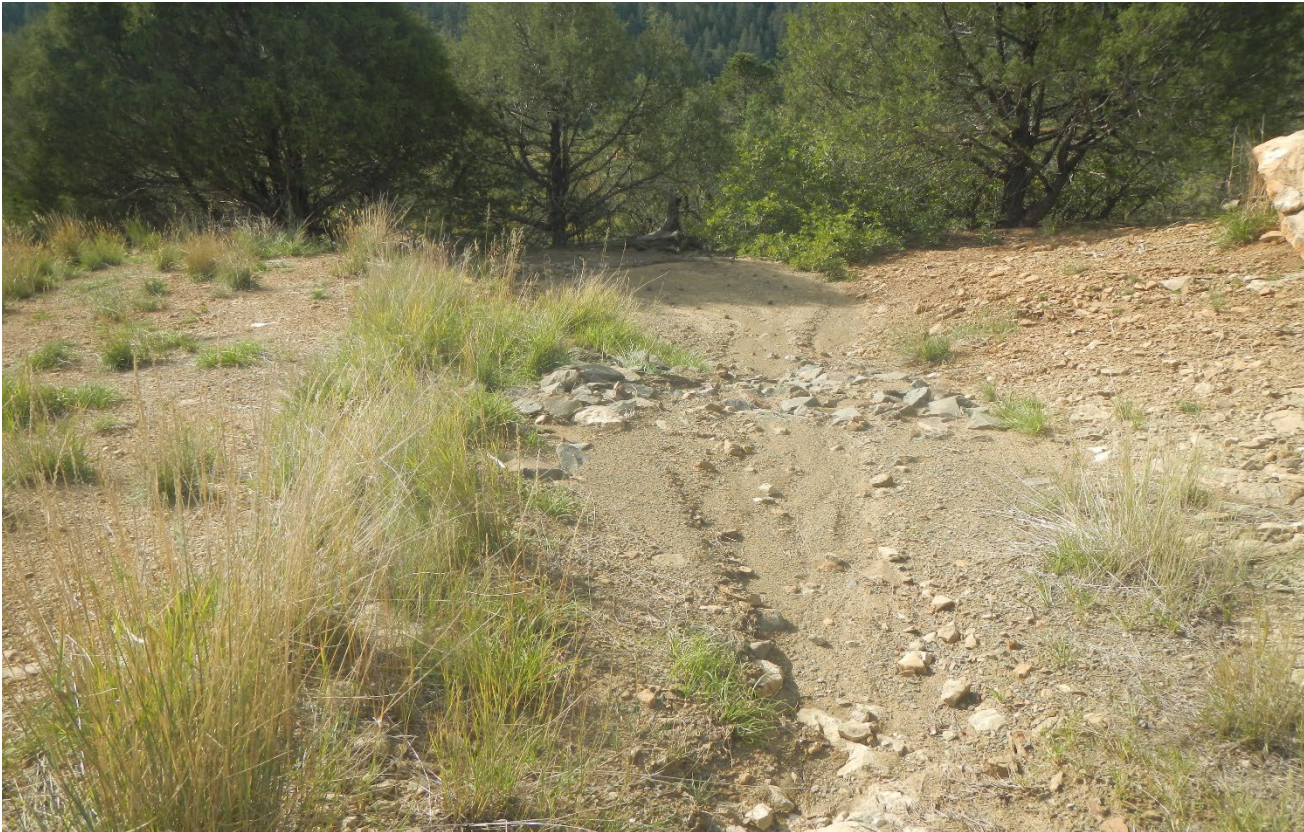
Photo 5. There is sediment accumulation along this rip/rap outlet which needs maintenance (shoveled/cleaned out).
