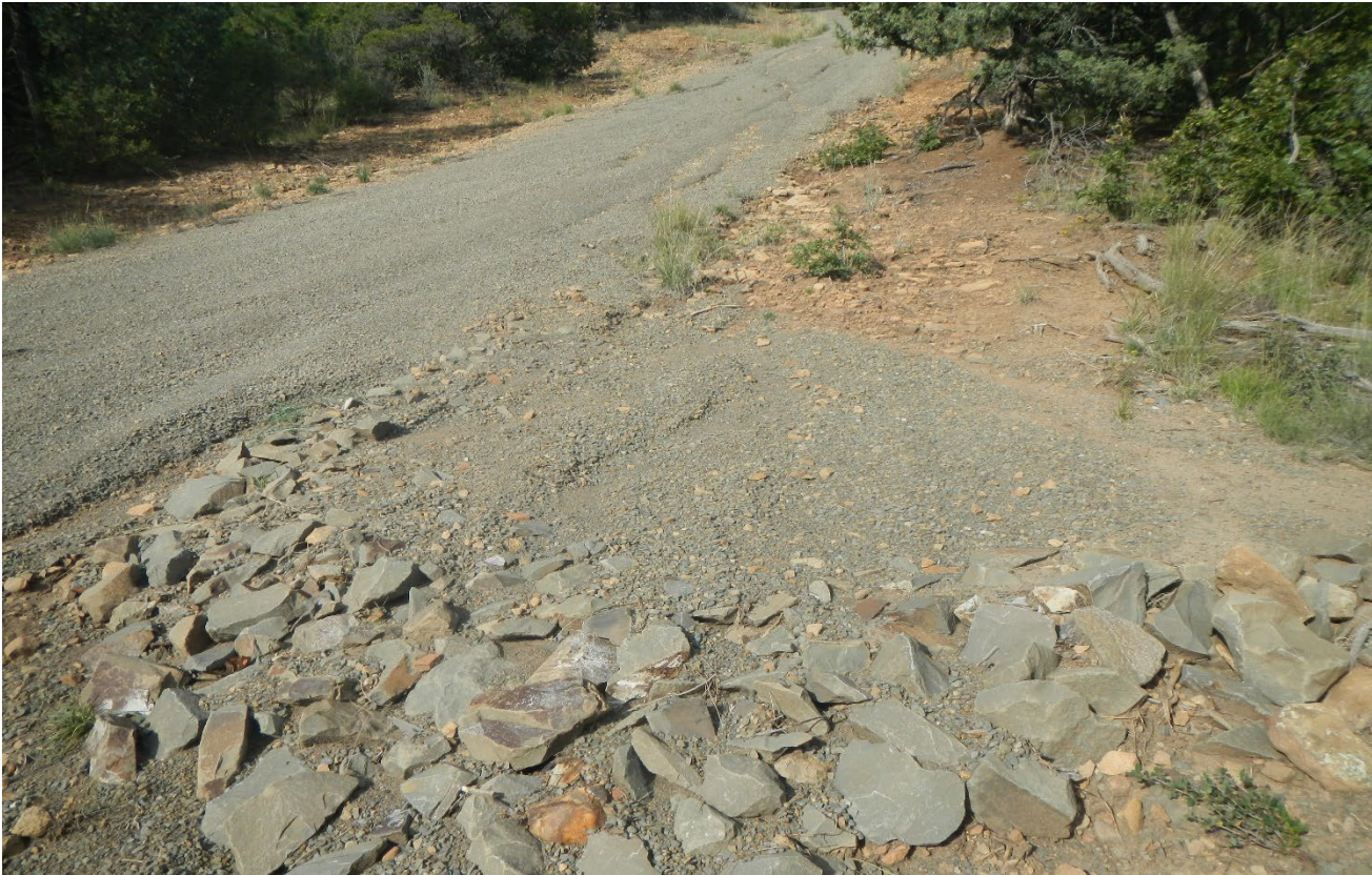
Photo 7. Facing west along the road. The rock check dams have filled in with gravel and sediment.
