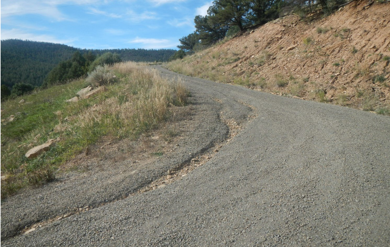
Photo 2. Facing southwest along the access road. There is an erosion channel down the road.
