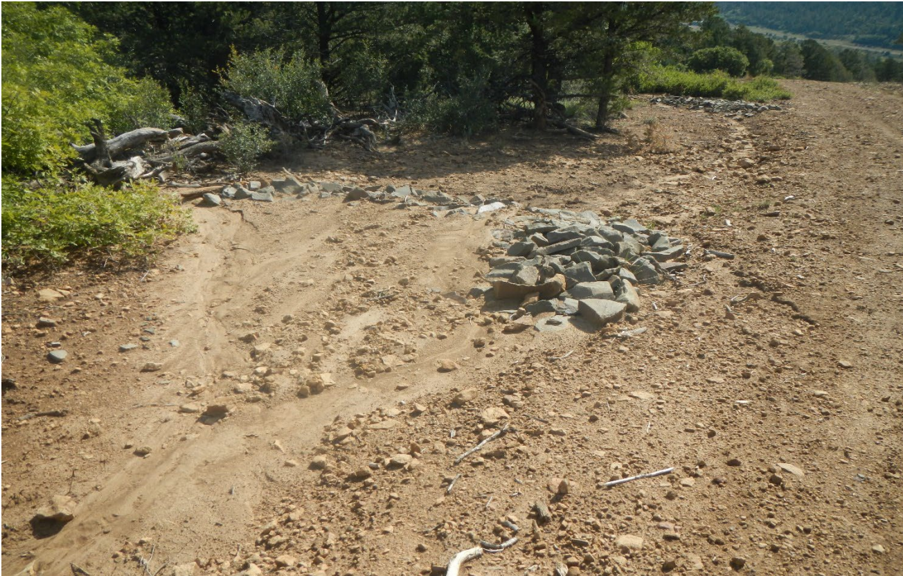
Photo 9. There is sediment accumulation along this rip/rap check dams which needs maintenance (shoveled/cleaned out).
