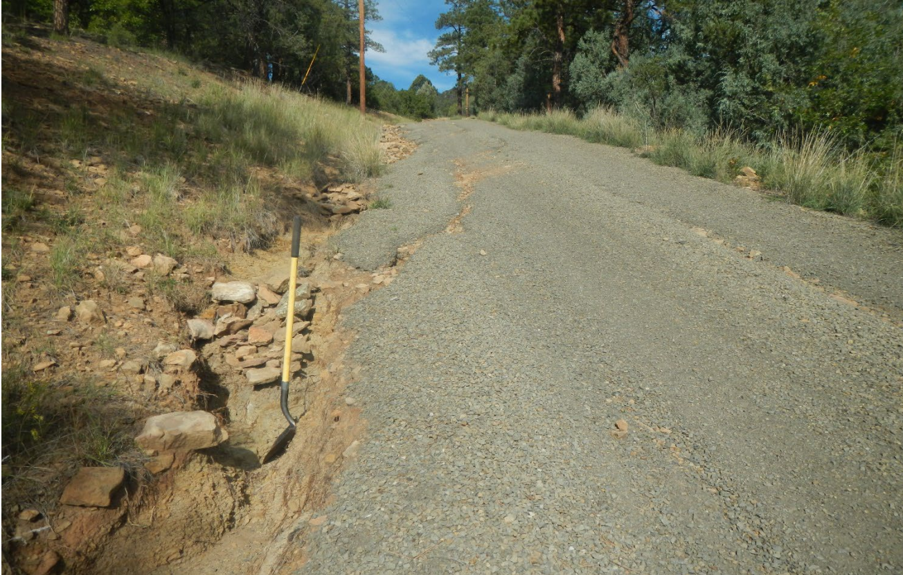
Photo 6. Facing northwest along the access road. There is erosion along the road side at this area. BMPs need to be installed to prevent further erosion.
