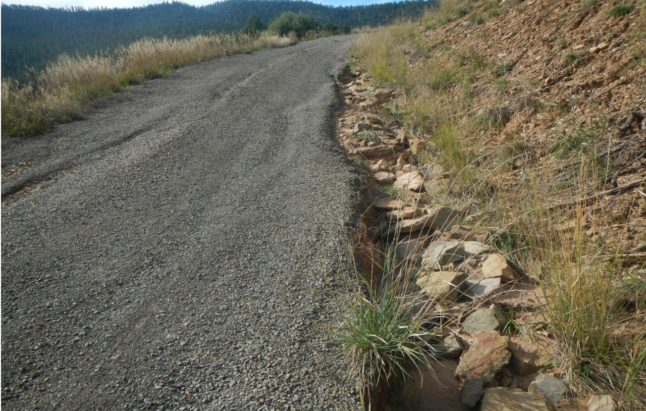
Photo 3. Facing southwest along the access road. Stormwater is cutting into the side of the road in this area. BMPs need to be installed to prevent further erosion.
