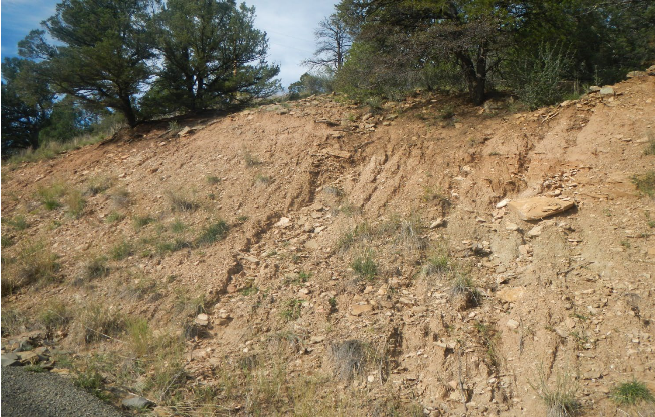
Photo 4. Stormwater run-on from the road that switches back above is causing erosion in this area along the road cut slope.
