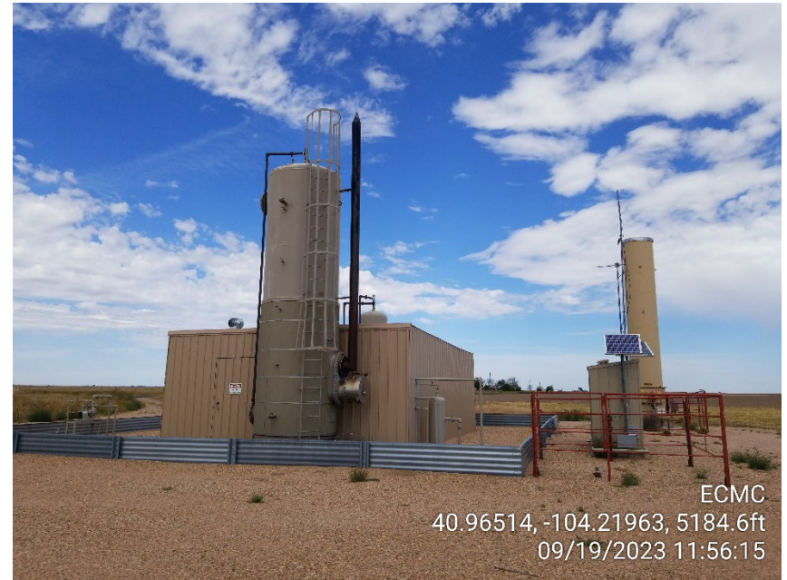
Photo 2 – Heater Treater, Gas Meter and ECD
