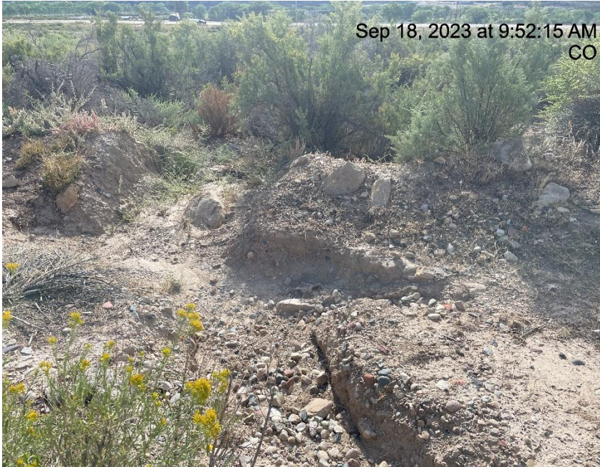
Photo # 9488 Erosion & transport of sediment off location & into a vegetated area/insufficient BMP's
