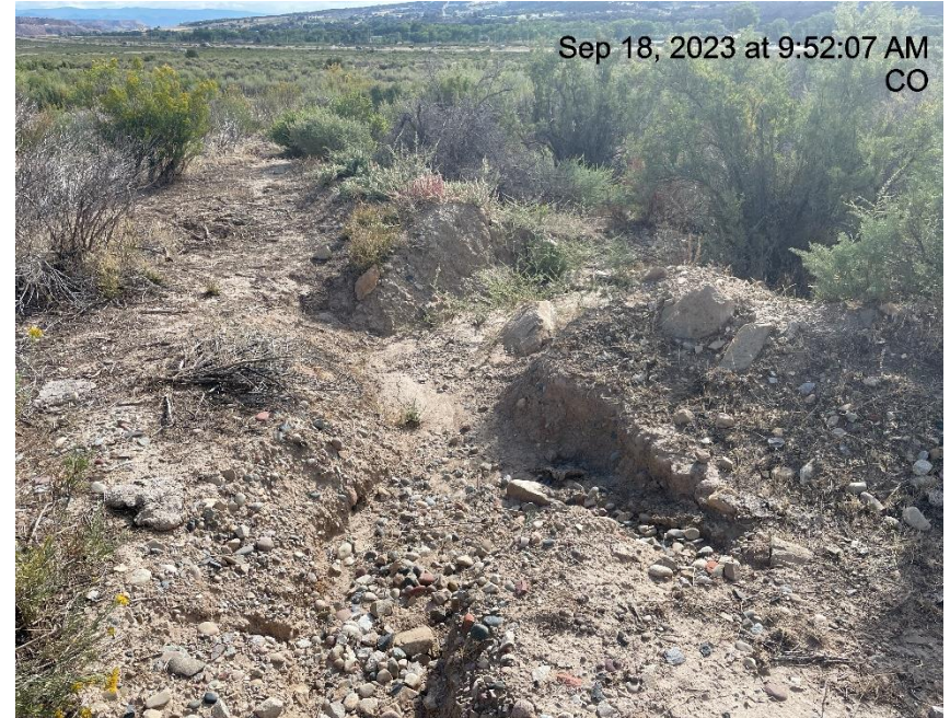
Photo # 9487 Erosion & transport of sediment off location & into a vegetated area/insufficient BMP's
